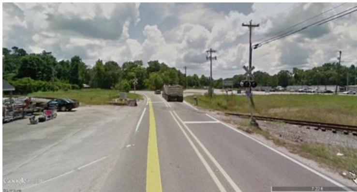
Figure 4.24: U.S. Highway 11 At-Grade Crossing (view looking southbound)
