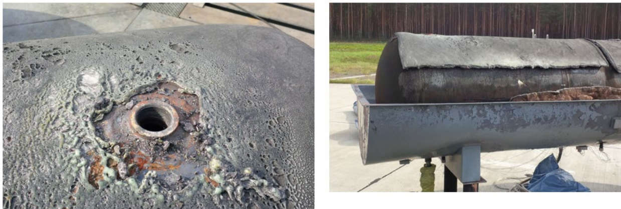
Figure 28. Test 1 – Images of Insulation Failure
