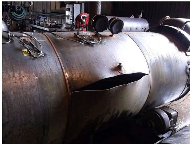
Figure 4. Burst Hydrostatic Tested Tank – Tensile Tear
