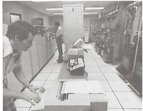
FIGURE 4. COMPUTER ROOM ON THE LOUISVILLE & NASHVILLE RAILROAD AT CORBIN, KENTUCKY
