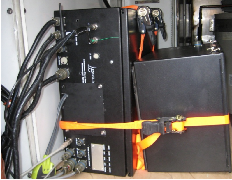
Figure 15: Stage 1 ATGMS Electronics on Amtrak Car 39000
