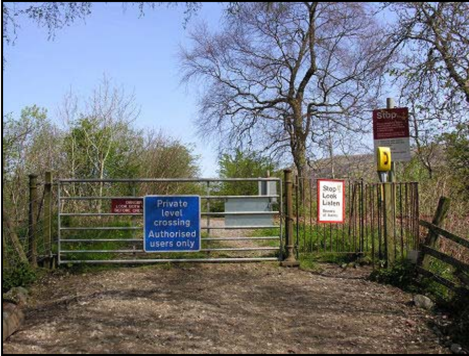
Figure 25. Private Highway-Rail Grade Crossing in Great Britain
