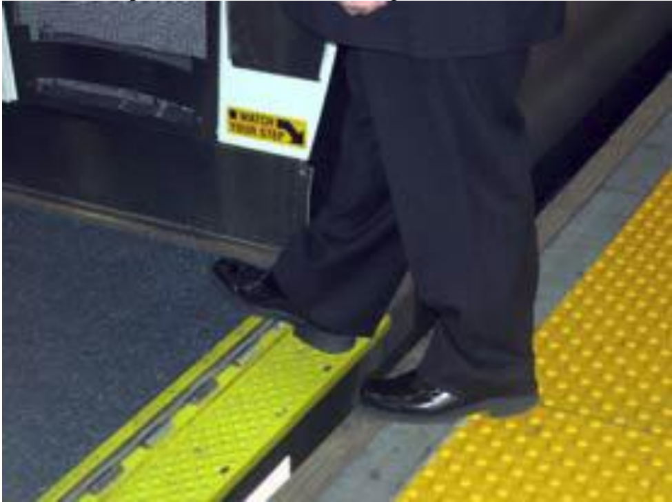
Photo 7. Example of Sacrificial Platform Edge and Retrofitted On-Borne Gap Extender (LIRR)
