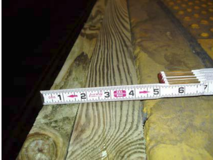
Photo 9. Example of Wood Platform Extender (LIRR)
