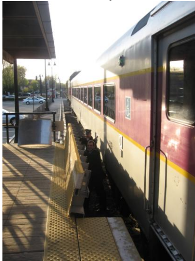
Photo 6. Manually-Lifted Station-Mounted Movable Ledge.
