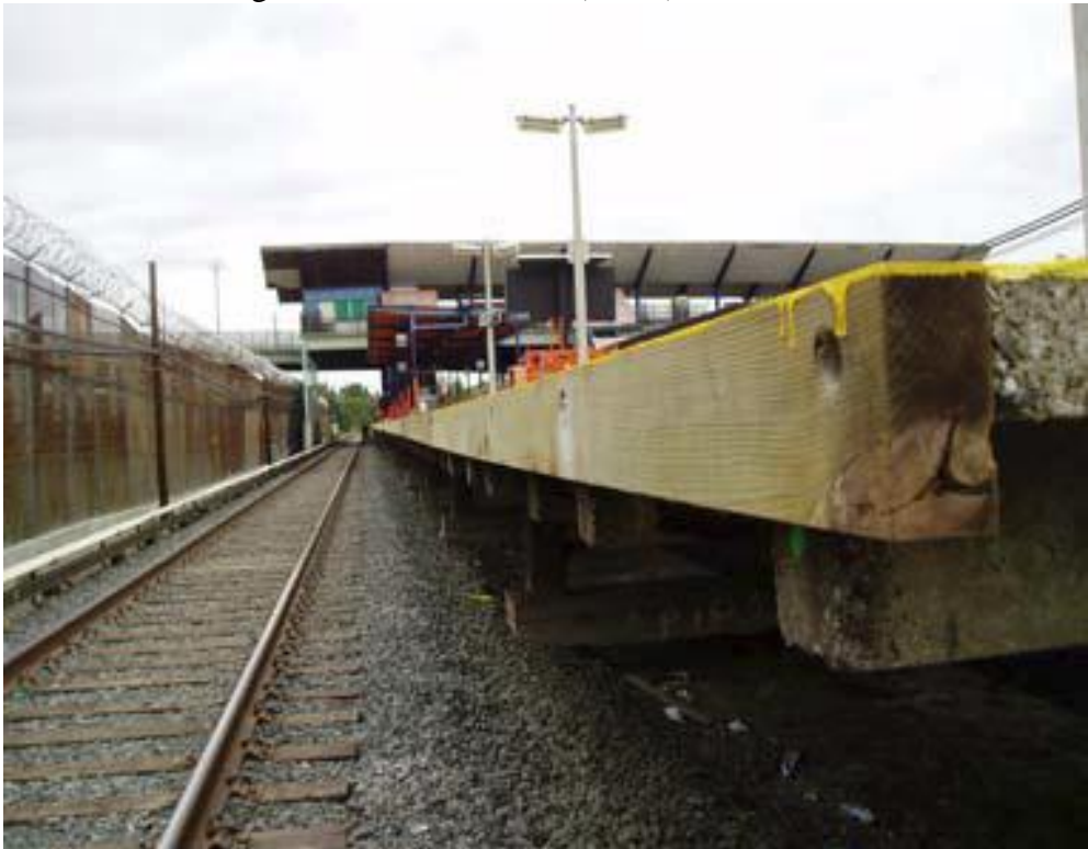
Photo 8. Extending Platform with Wood (LIRR)
