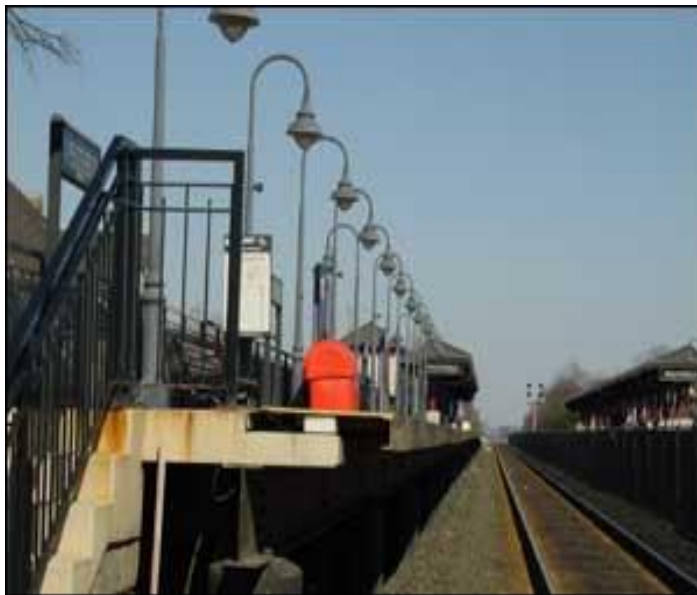
Photo 5. Platform Mounted Mechanical Extender.
