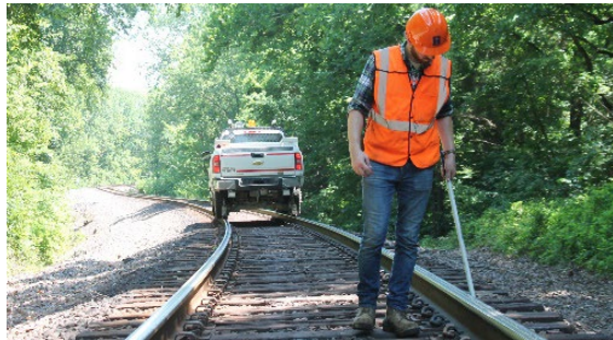
Figure 4. Spike inspection methods involve walking curves and tapping each spike
