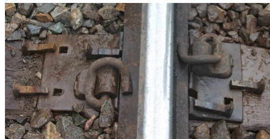
Figure 1. Premium elastic fastener with five broken spikes
