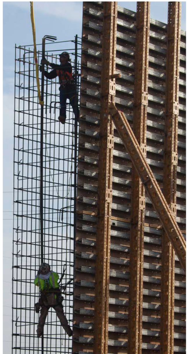
PHOTO: CENTRAL VALLEY CONSTRUCTION WORKERS INSTALLING STEEL REBAR
