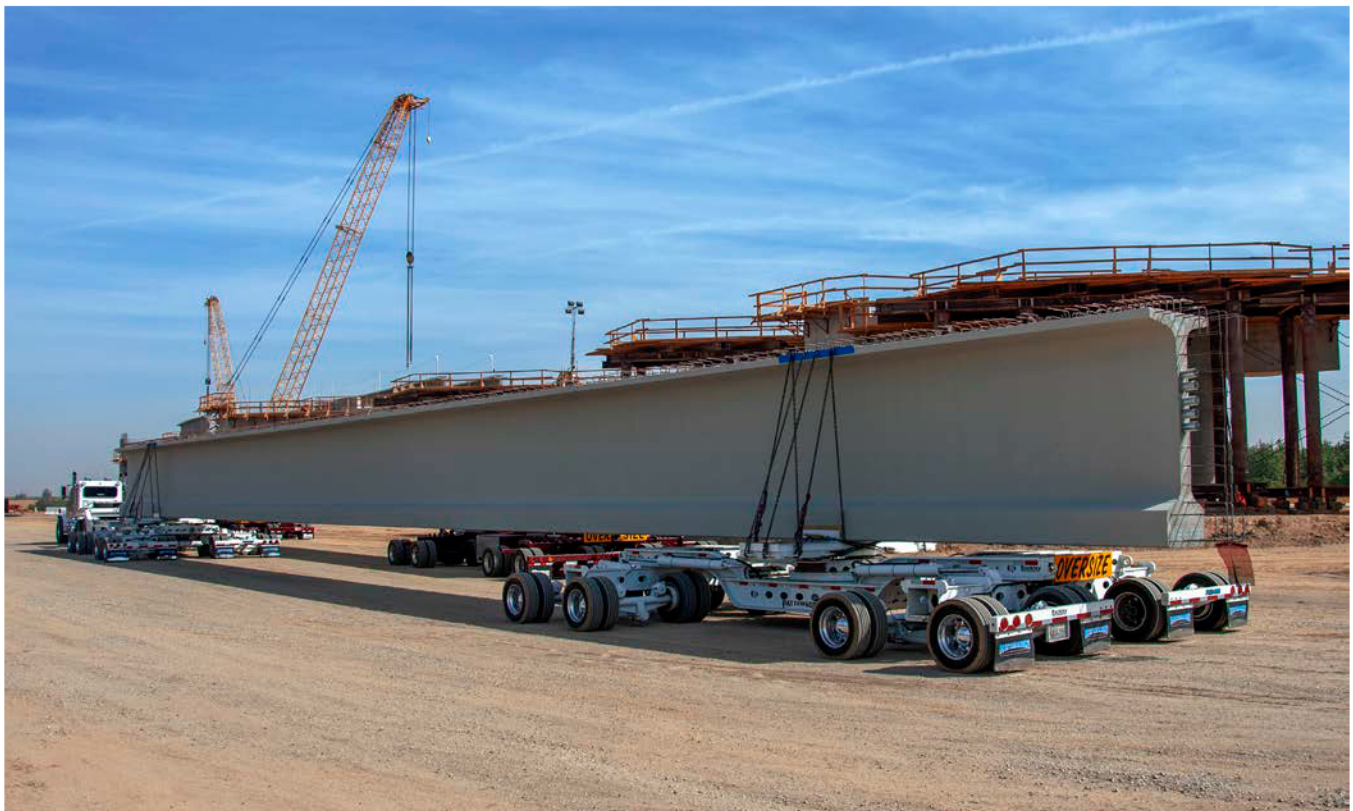
PHOTO: THE ROAD 27 OVERCROSSING WILL BE OVER 700 FEET LONG WITH THE LONGEST SPAN STRETCHING 198 FEET.
