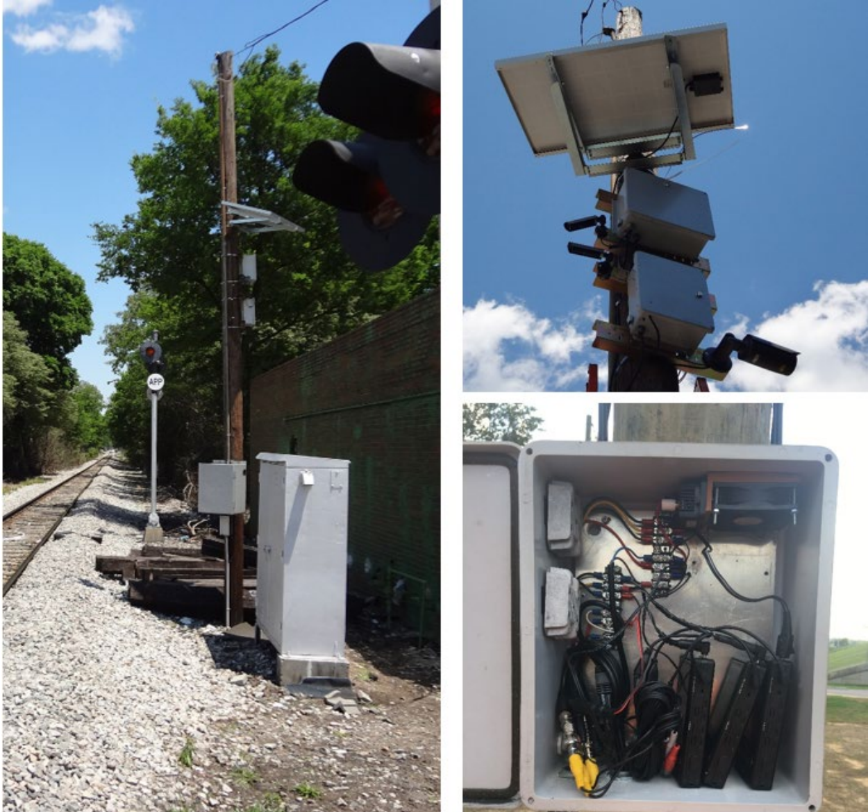
Figure 8. Baseline Video Data Collection Systems in Collegeville, AL
