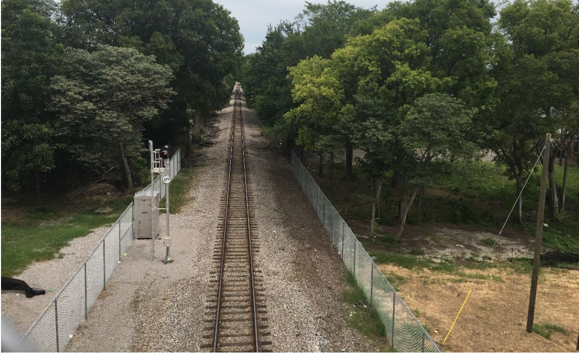
Figure 7. Railroad ROW to East of the Overpass Bridge
