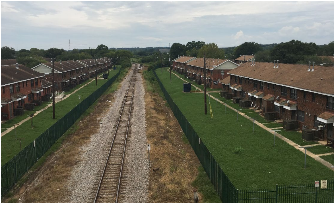
Figure 6. Railroad ROW to West of the Overpass Bridge
