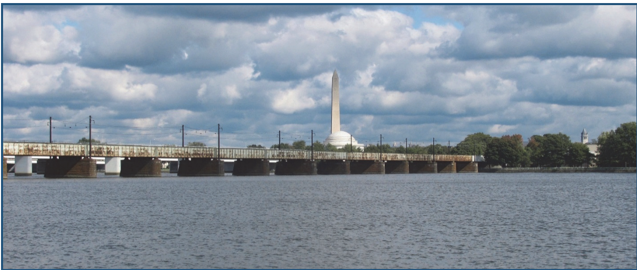
Long Bridge over the Potomac River
