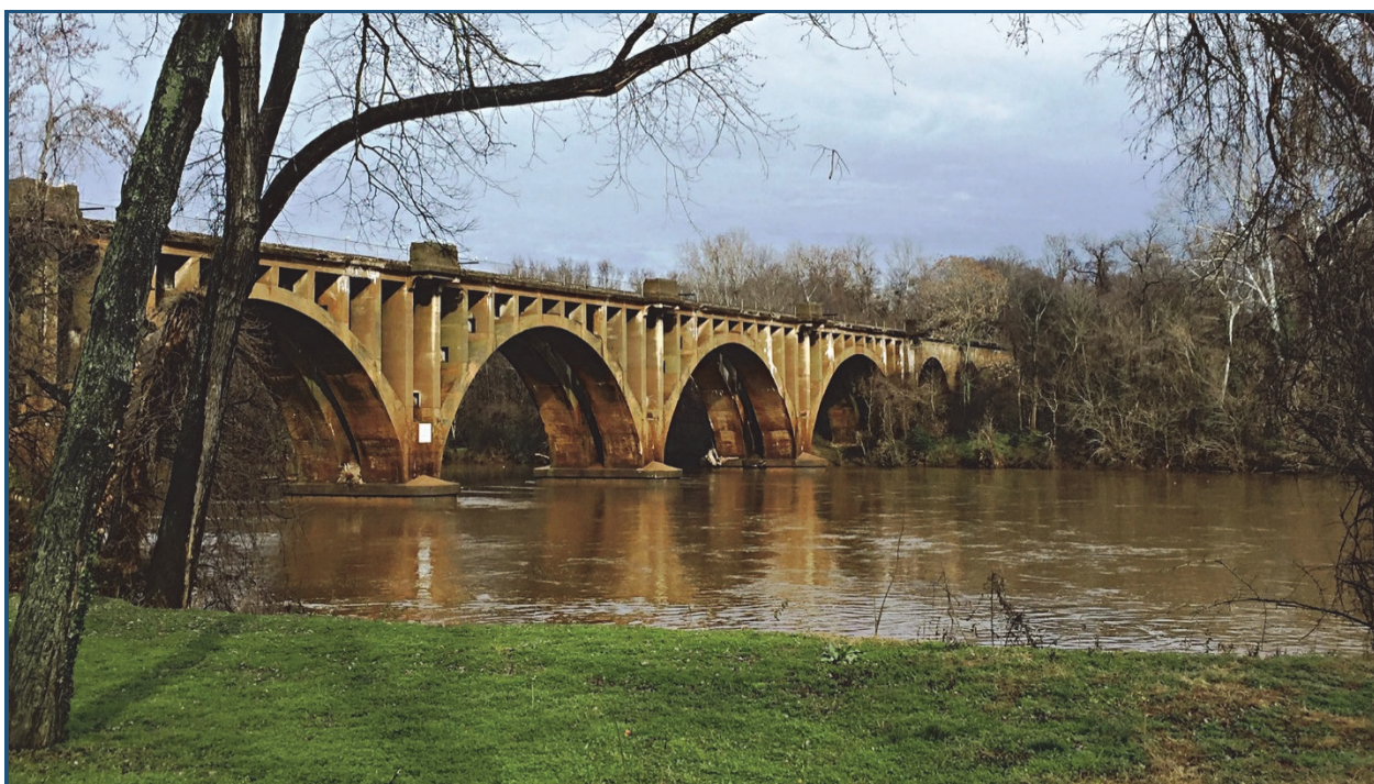
Rail Bridge over the Rappahannock River in Area 3 (Fredericksburg)
