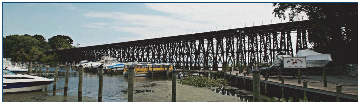
Rail Bridge over Neabsco Creek in Area 2 (Northern Virginia)
