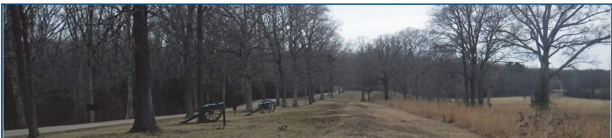
Earthwork/Jackson’s Earthwork (Area 3, Fredericksburg)
