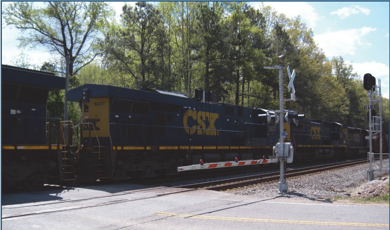
Vaughan Road Existing At-Grade Crossing (Area 5, Ashland)
