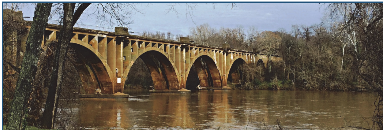
Rappahannock River Railroad Bridge (Area 3, Fredericksburg)
