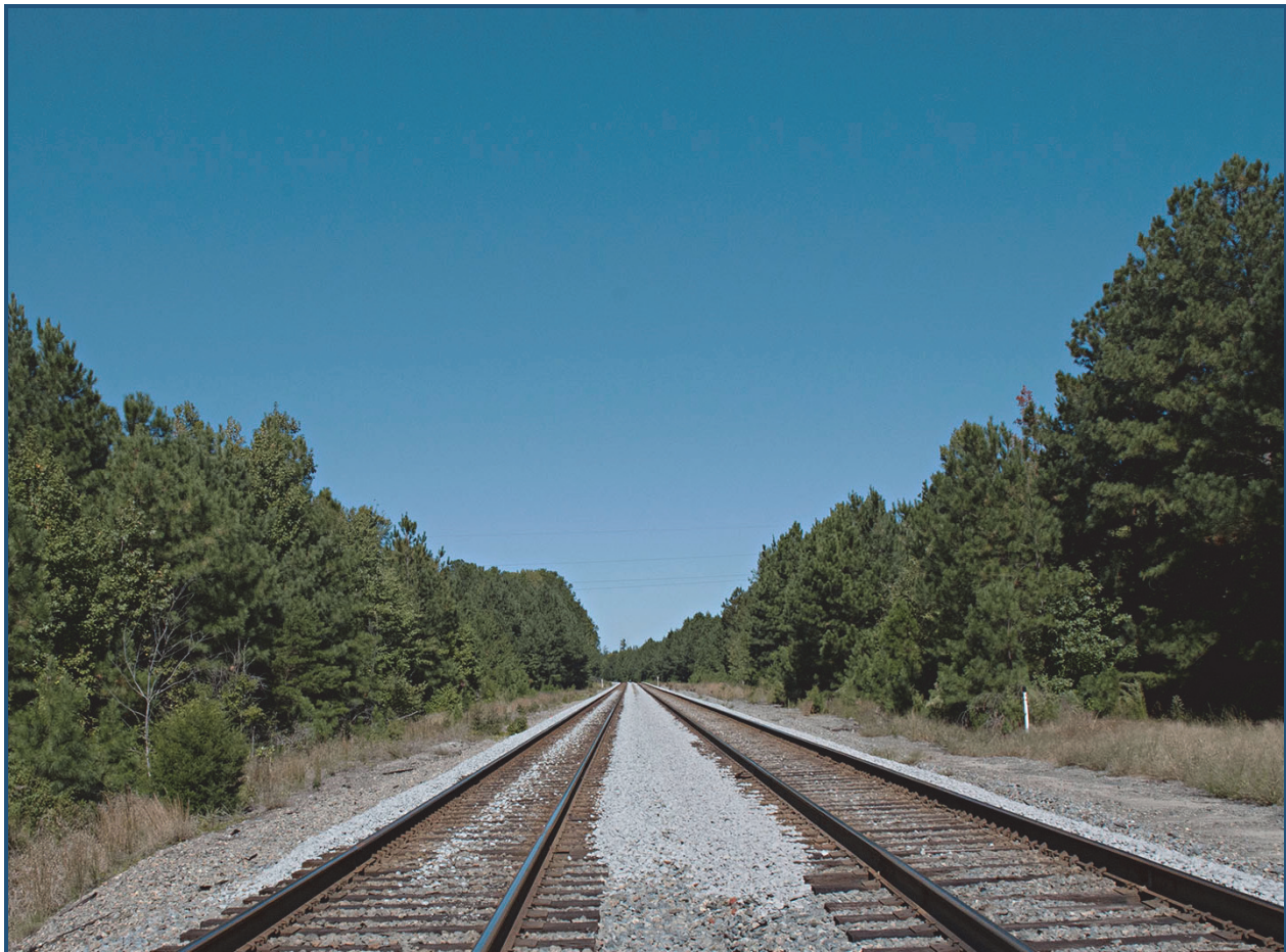
Existing DC2RVA Rail Corridor
