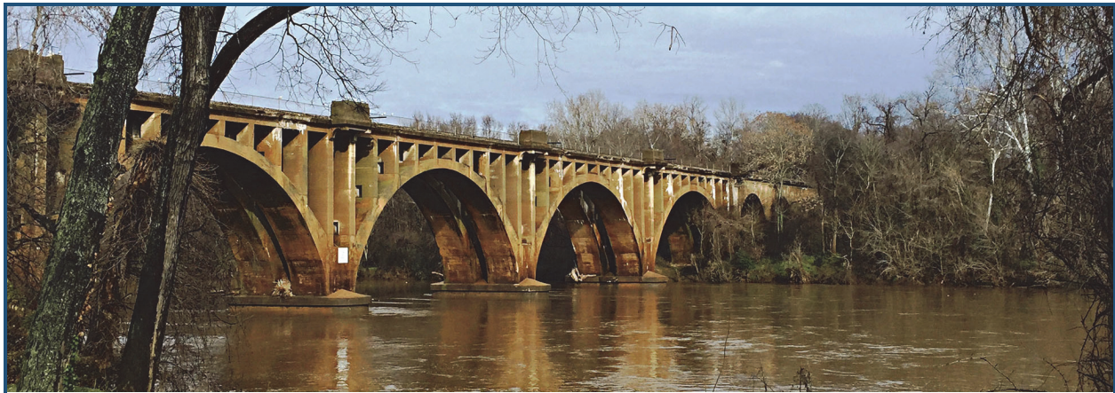
Rappahannock River Railroad Bridge (Area 3, Fredericksburg)
