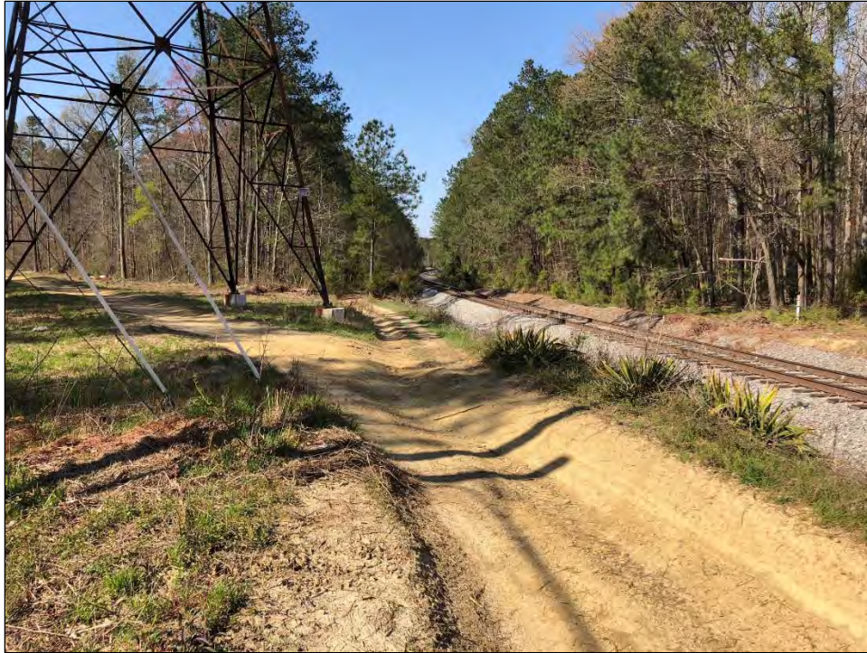
FIGURE 4-219: UTILITY AND RAIL CONSTRUCTION DISTURBANCE ALONG CSXT CORRIDOR IN AREA 6H, LOOKING SOUTH
