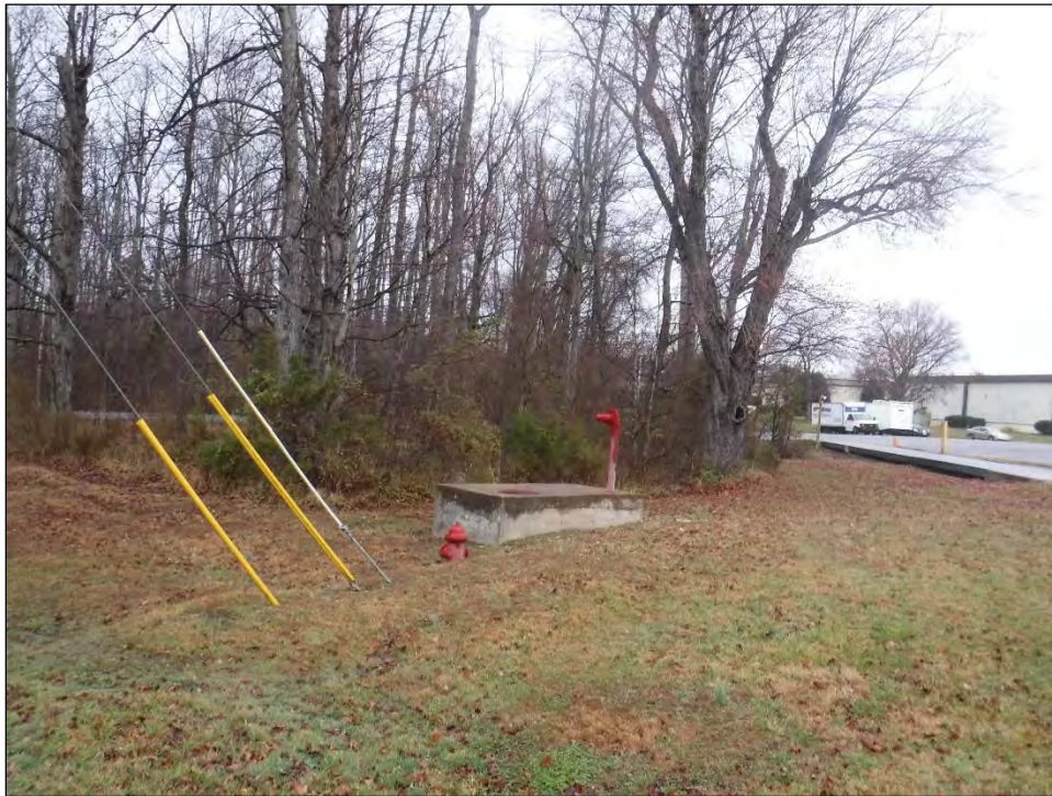
FIGURE 4-88: BURIED UTILITY DISTURBANCE IN AREA 3C, LOOKING WEST
