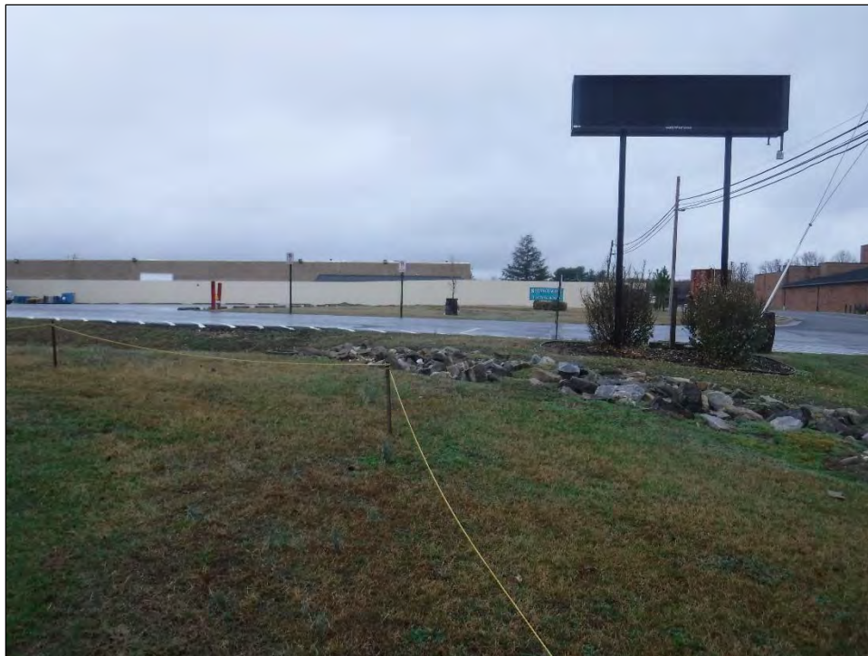
FIGURE 4-79: REPRESENTATIVE VIEW OF AREA 3 SETTING, LOOKING NORTHEAST
