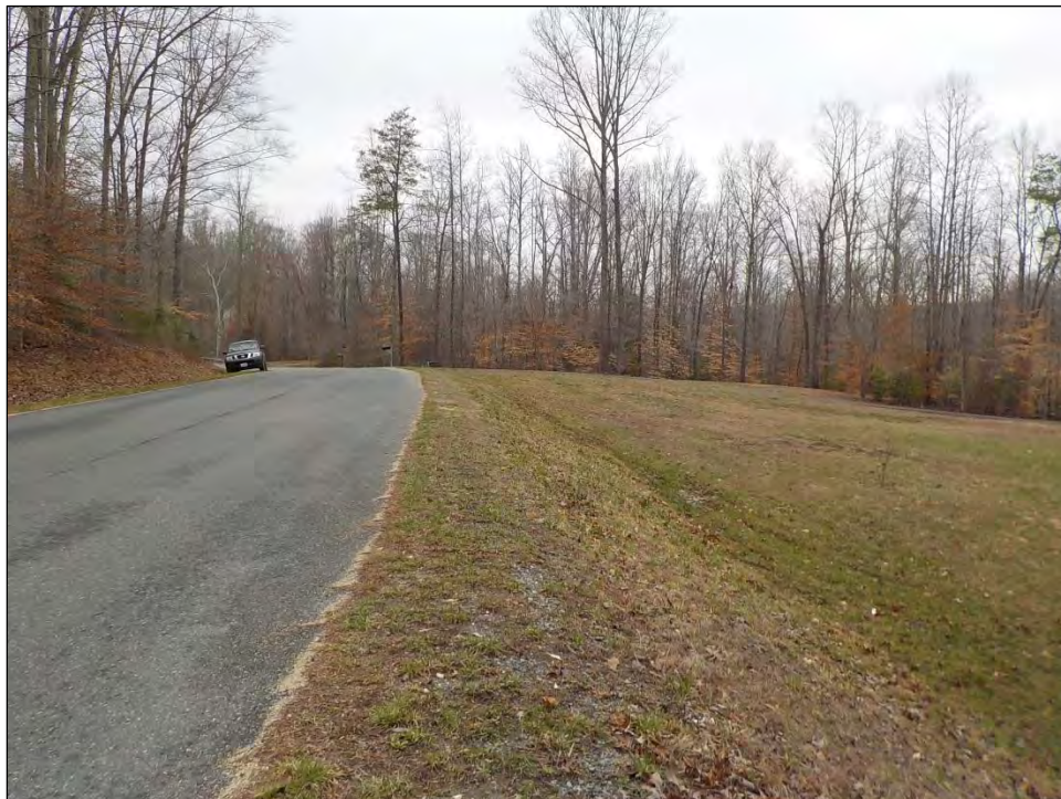
FIGURE 4-40: DISTURBANCE FROM ROAD GRADING IN AREA 21, LOOKING SOUTH
