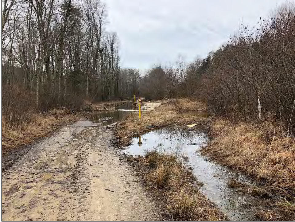
FIGURE 4-99: ROAD AND BURIED UTILITY DISTURBANCE IN AREA 3F, LOOKING SOUTH
