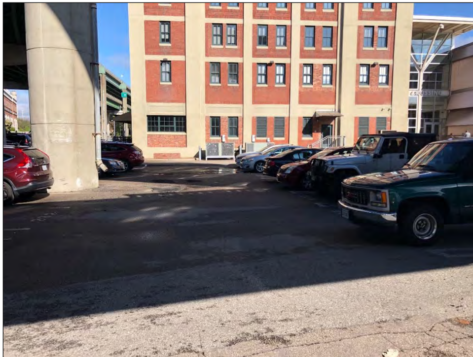
FIGURE 4-227: OVERVIEW OF SITE 44HE1094, LOOKING WEST
