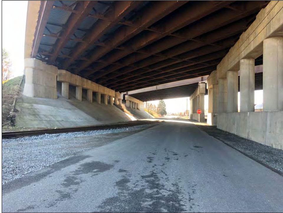
FIGURE 4-195: AREA 6C ALONG CSXT RAIL, LOOKING SOUTH
