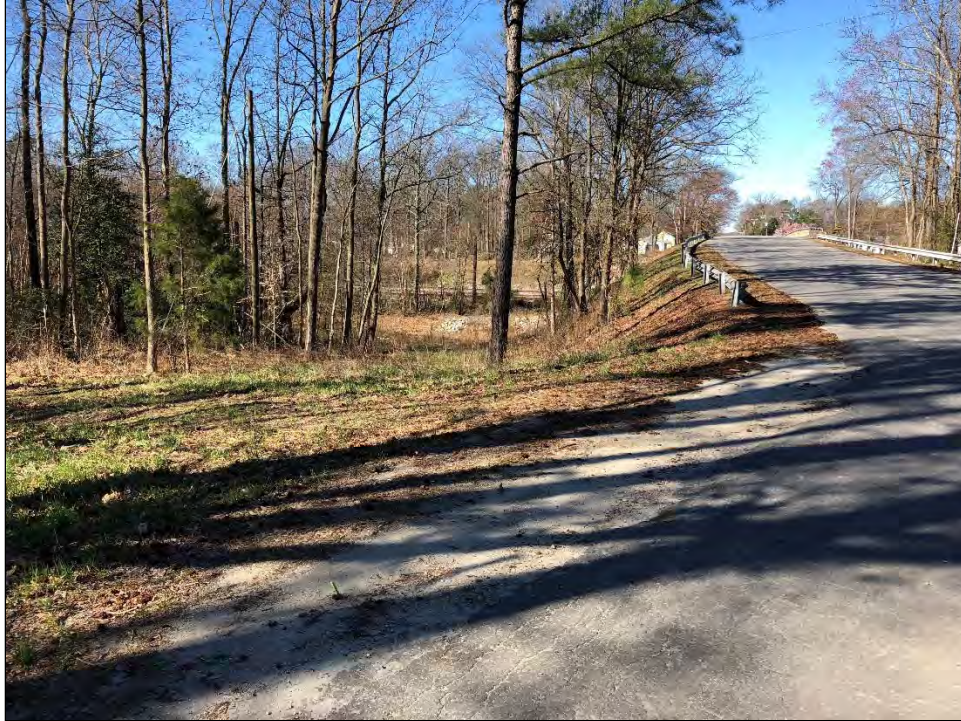
FIGURE 4-212: GRADING OF OVERPASS IN AREA 6G ON ELLIHAM AVENUE, LOOKING WEST
