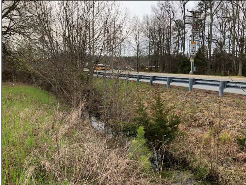
FIGURE 4-166: ROAD CONSTRUCTION DISTURBANCE IN AREA 5B, LOOKING EAST
