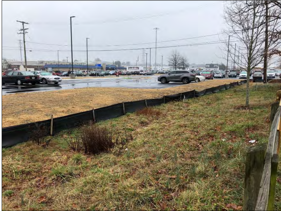
FIGURE 4-191: AMTRAK STATION CONSTRUCTION DISTURBANCE IN AREA 6B, LOOKING SOUTHEAST
