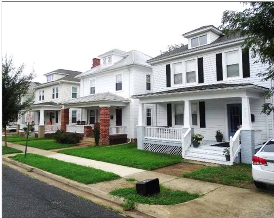
FIGURE 3-108: VIEW OF SEVERAL FOURSQUARE HOUSES ALONG THE 800 BLOCK OF CHARLOTTE STREET, LOOKING EAST
