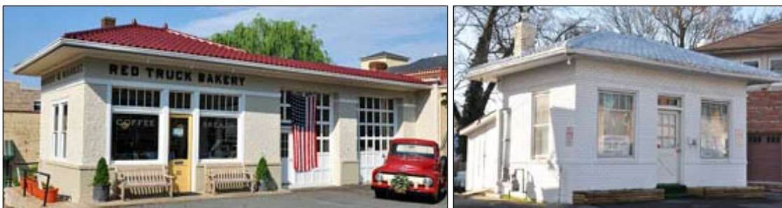
FIGURE 3-98: TWO EARLY TWENTIETH CENTURY, MISSION REVIVAL-STYLED GAS STATIONS IN WARRENTON (LEFT) AND WINCHESTER (RIGHT), VIRGINIA (ROADSIDEARCHITECTURE.COM N.D.)
