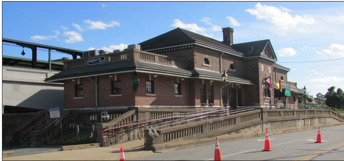
FIGURE 3-45: FREDERICKSBURG TRAIN STATION (111-0132-0704), NORTHEAST OBLIQUE
