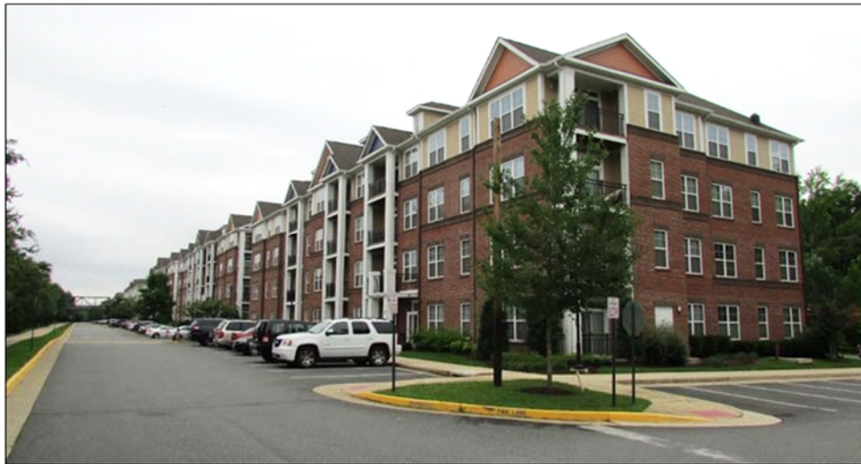
FIGURE 3-116: OVERVIEW OF APARTMENTS AT COBBLESTONE SQUARE AT 627 COBBLESTONE CIRCLE, LOOKING EAST
