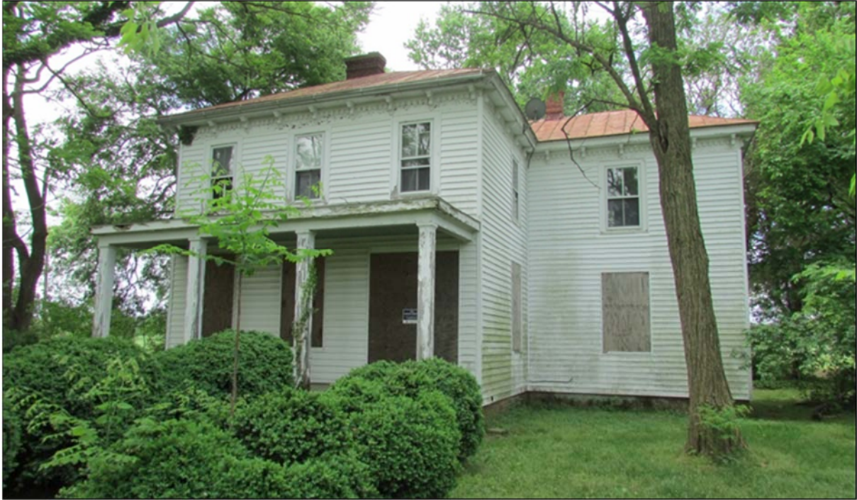
FIGURE 3-123: SLAUGHTER PEN FARM, VIEW OF FAÇADE OR NORTHEAST ELEVATION
