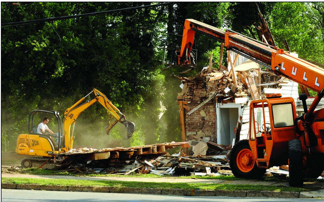
FIGURE 3-33: THE HOUSE DURING DEMOLITION (FREDERICKSBURG FREE LANCE-STAR 2015)
