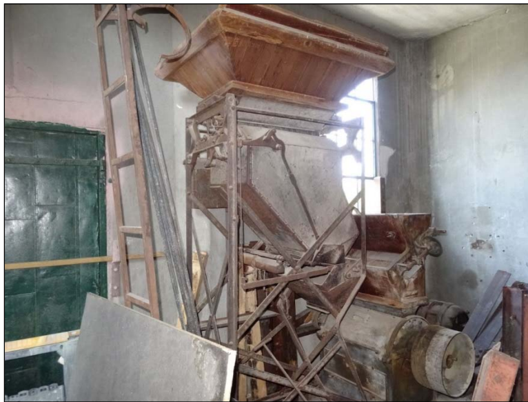
FIGURE 3-70: PART OF THE ORIGINAL MACHINERY IN THE GRAIN ELEVATOR
