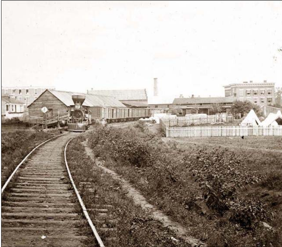
FIGURE 3-154: SECTION OF O&A RAILROAD IN MANASSAS (O'SULLIVAN 1862)
