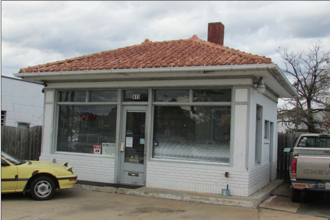
FIGURE 3-93: PRIMARY (SOUTH) ELEVATION OF THE FORMER FILLING STATION AT 411 LAFAYETTE BOULEVARD
