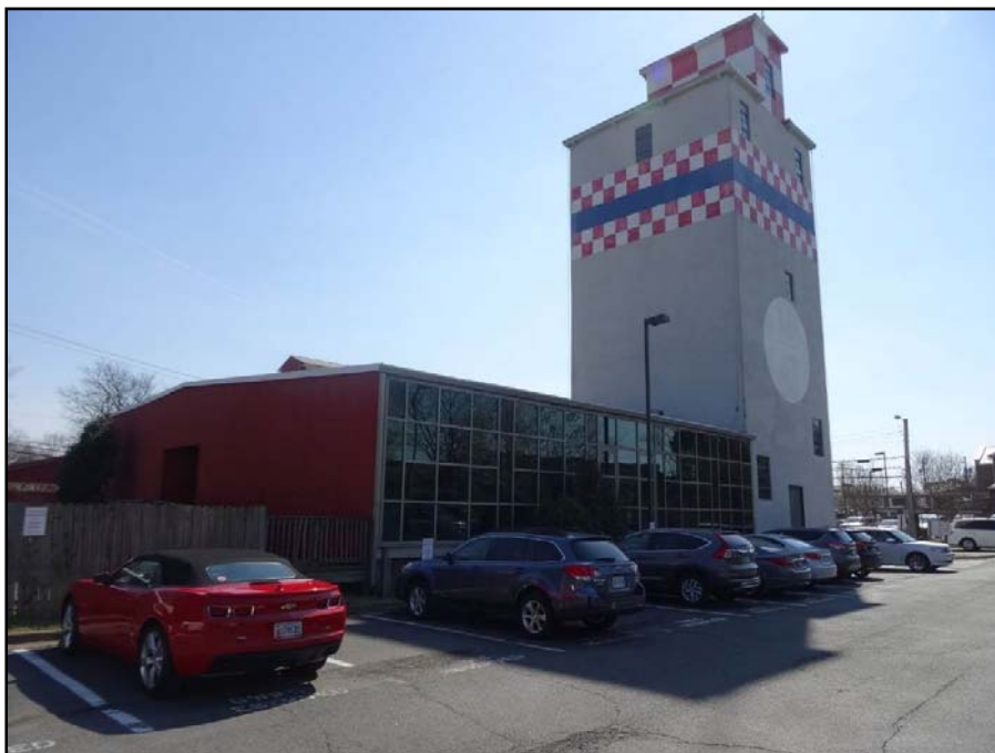
FIGURE 3-62: NORTHEAST OBLIQUE VIEW OF PURINA TOWER COMPLEX
