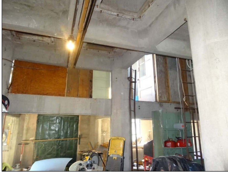
FIGURE 3-69: INTERIOR OF GRAIN ELEVATOR TOWER, LOOKING WEST-NORTHWEST
