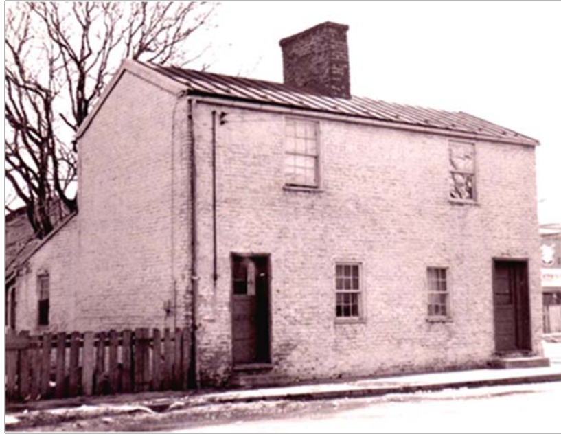
FIGURE 3-78: NORTHEAST OBLIQUE VIEW OF 314-316 FREDERICK STREET TAKEN IN 1958 (HFFI N.D.)
