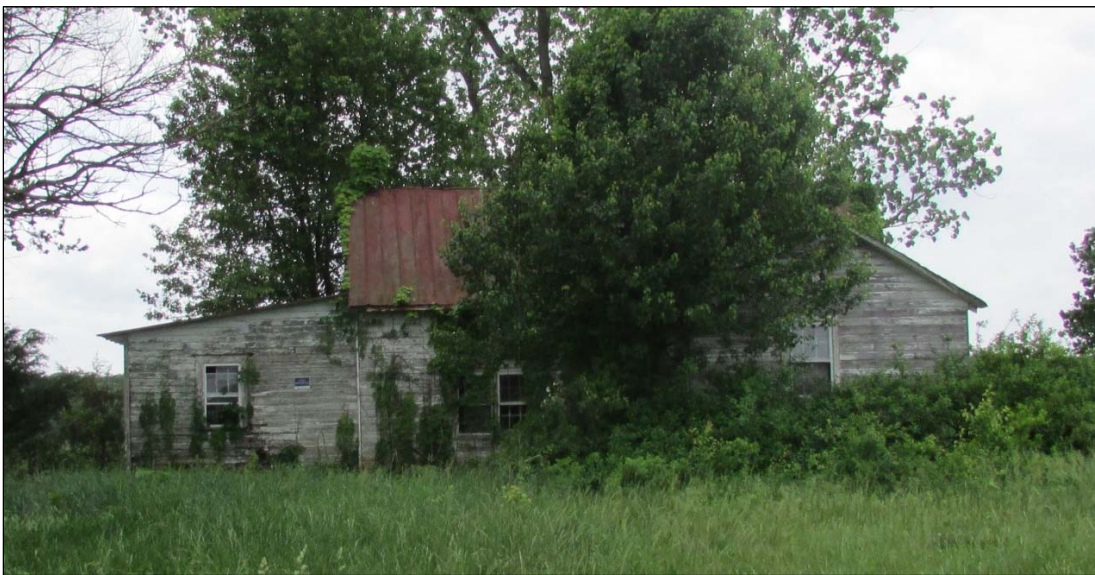
FIGURE 3-130: NORTHEAST OR REAR ELEVATION OF TENANT HOUSE
