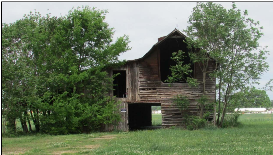
FIGURE 3-128: SLAUGHTER PEN FARM, SOUTHEAST ELEVATION OF BARN
