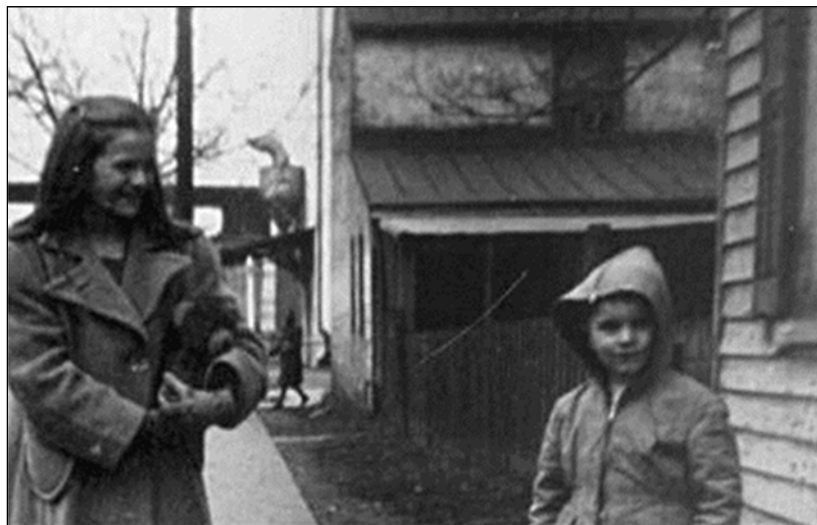
FIGURE 3-79: 1949 PHOTO SHOWING REAR (SOUTH) ELEVATION OF 316 FREDERICK STREET, LOOKING NORTH ALONG CHARLES STREET (STROBEL 2015). NOTE: THE REAR OF GEORGE ALER HOUSE, 314-316 FREDERICK STREET IS VISIBLE IN BACKGROUND.
