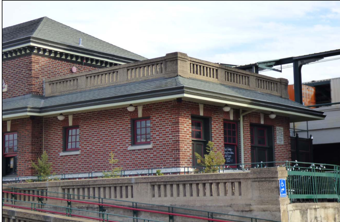
FIGURE 3-46: FREDERICKSBURG TRAIN STATION, NORTHWEST OBLIQUE OF CIRCA-1927 WEST WING
