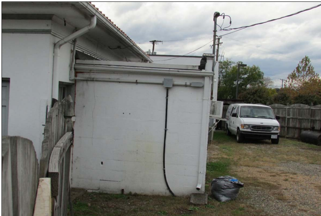
FIGURE 3-95: ONE-STORY, CONCRETE-BLOCK REAR (NORTH) ADDITION
