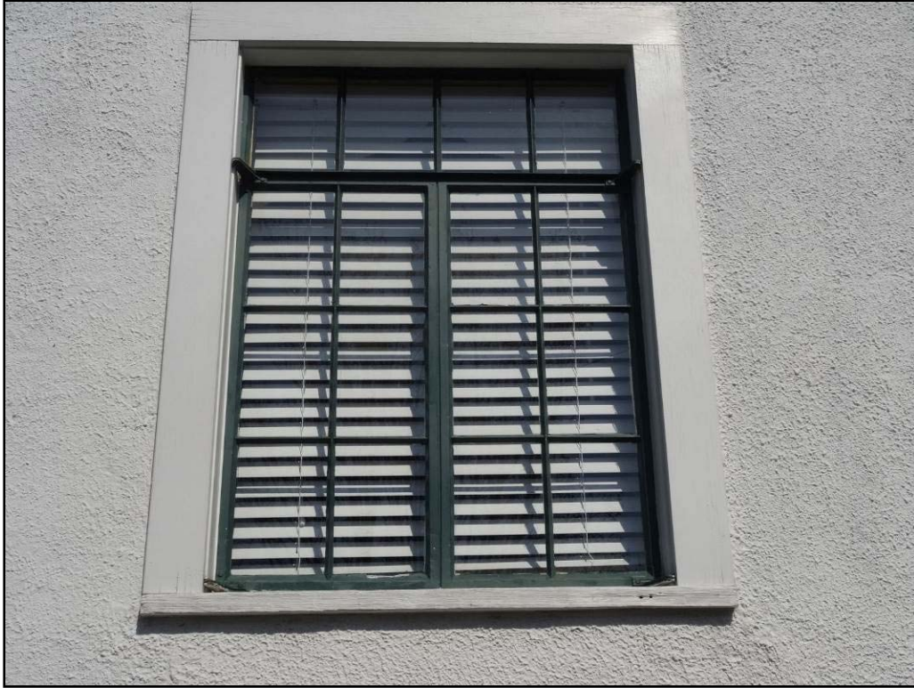
FIGURE 3-64: DETAIL VIEW OF METAL CASEMENT WINDOW
