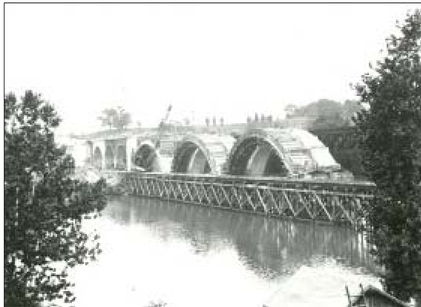
FIGURE 3-15: PHOTOGRAPH OF THE RAPPAHANNOCK RIVER RAILROAD BRIDGE UNDER CONSTRUCTION IN 1926 (BLACKWELL 2016)
