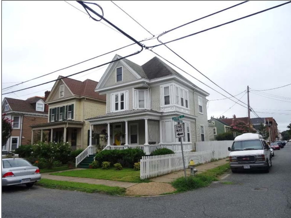
FIGURE 3-107: VIEW OF QUEEN ANNE-STYLE DWELLINGS ON THE SOUTHWEST CORNER OF LEWIS AND WINCHESTER STREETS, LOOKING SOUTHEAST
