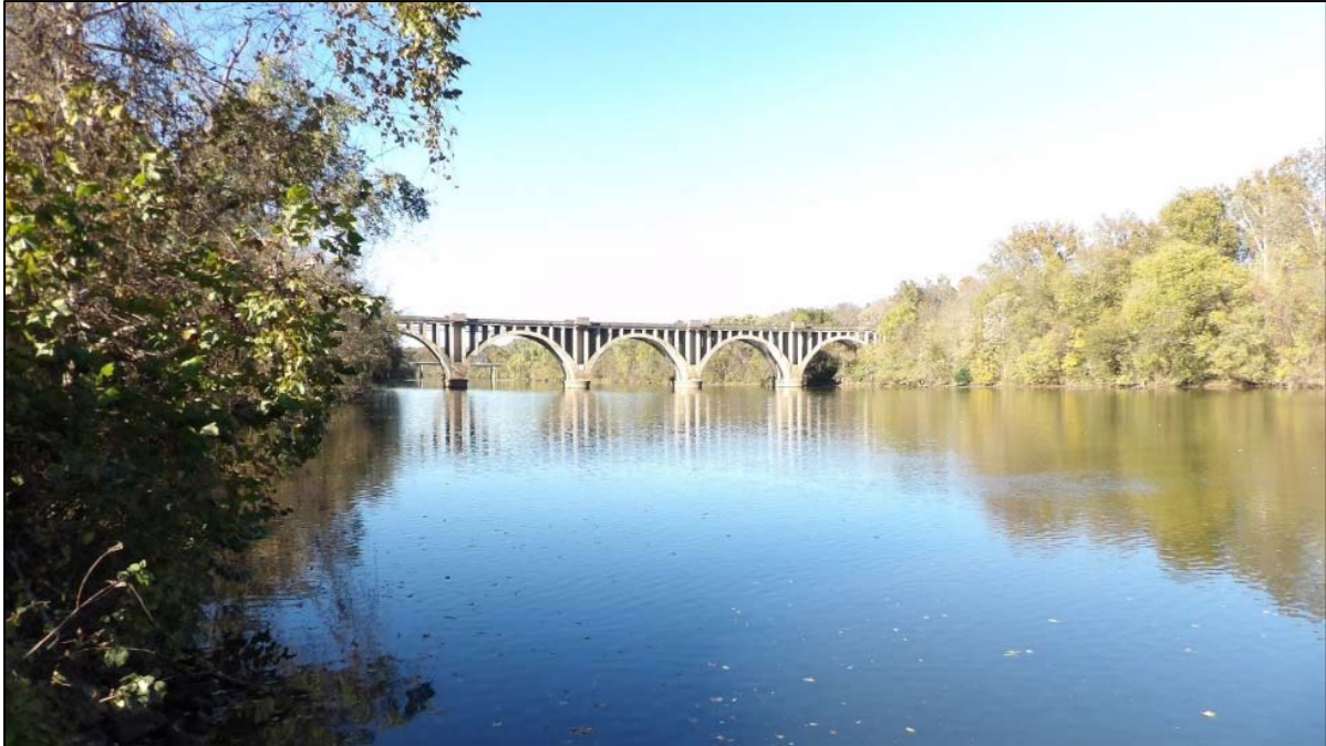
FIGURE 3-19: VIEW OF RAPPAHANNOCK RIVER RAILROAD BRIDGE, LOOKING NORTHWEST FROM CITY DOCK
