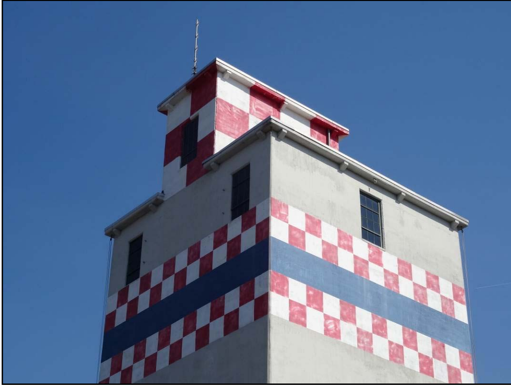
FIGURE 3-65: CLOSE-UP VIEW OF GRAIN ELEVATOR ROOF AND CUPOLA OF PURINA TOWER
