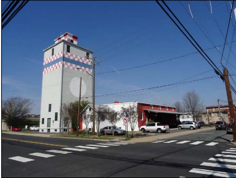
FIGURE 3-61: SOUTHWEST OBLIQUE VIEW OF PURINA TOWER COMPLEX
