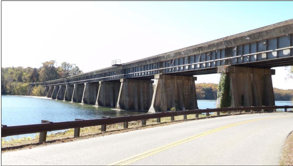
FIGURE 3-172: THE CIRCA-1945 AQUIA CREEK BRIDGE (500-0001-0028)
