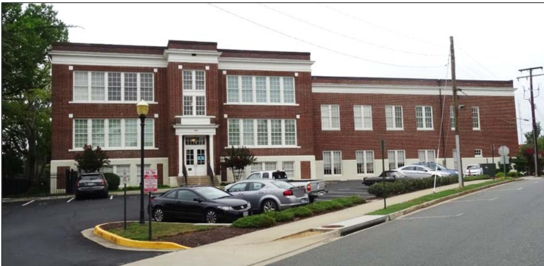
FIGURE 3-114: EAST ELEVATION OF THE MATTHEW FONTAINE MAURY SCHOOL AT 900 BARTON STREET (111-0009-0014)
