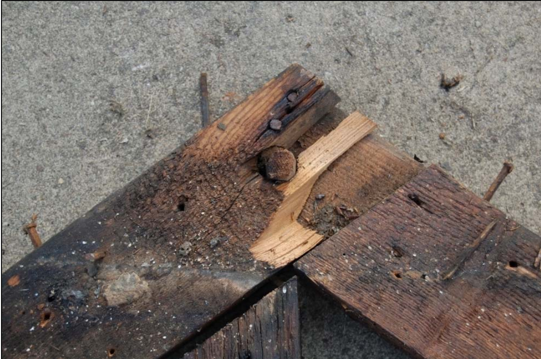
FIGURE 3-34: SAMPLE OF FRAMING AND FASTENERS FROM THE 1843 CORE (CUMMINGS 2015)
