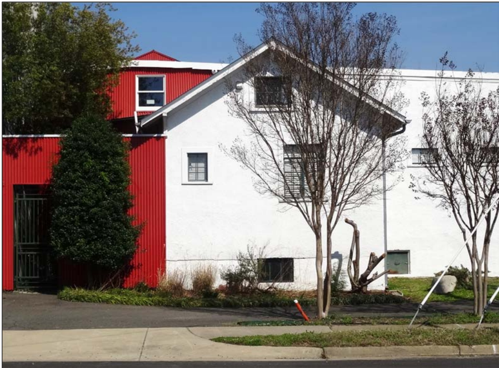
FIGURE 3-63: WEST ELEVATION OF THE ONE-STORY ADDITION ON WEST ELEVATION OF WAREHOUSE BLOCK AT PURINA TOWER COMPLEX
