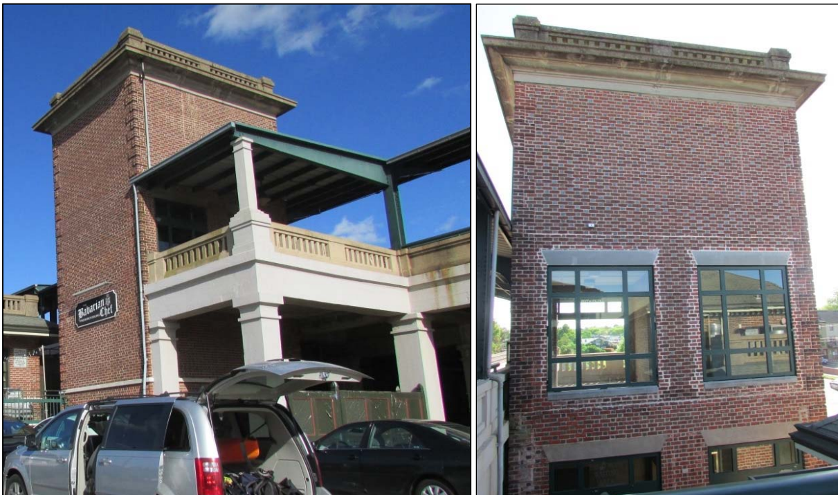
FIGURE 3-49: NORTHWEST OBLIQUE AT LEFT AND EAST ELEVATION OF FREIGHT TOWER
