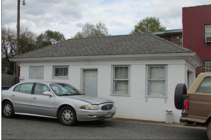
FIGURE 3-96: SOUTHEAST OBLIQUE VIEW OF THE CIRCA-1940, ONE-STORY GARAGE
