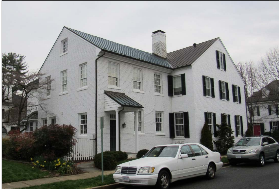
FIGURE 3-15: CIRCA-1990 ADDITION, SOUTH OBLIQUE
