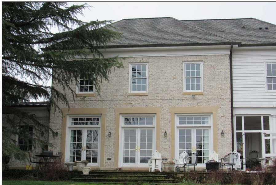
FIGURE 3-26: NORTHEAST ELEVATION OF ADDITION
