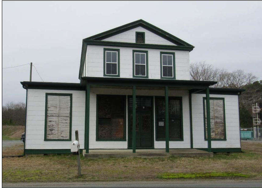
FIGURE 3-152: COBBS STORE (042-0341), NORTHEAST ELEVATION
