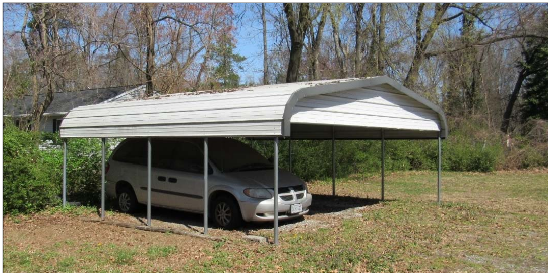
FIGURE 3-105: CARPORT, LOOKING NORTH
