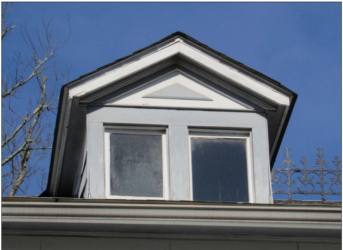
FIGURE 3-135: DETAIL OF DORMER
