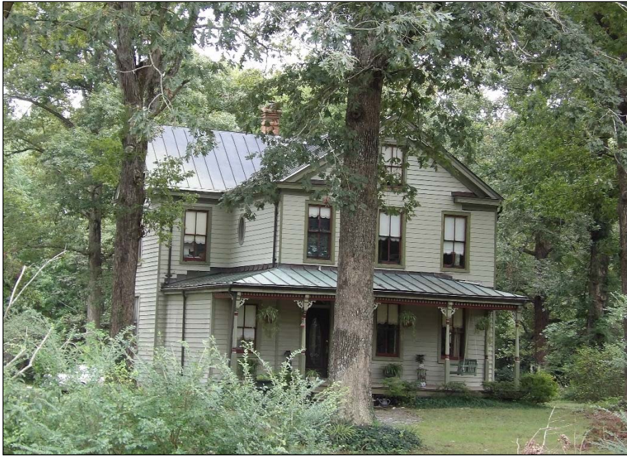
FIGURE 3-164: HOUSE AT 11531 MILL ROAD, NORTHEAST OBLIQUE
