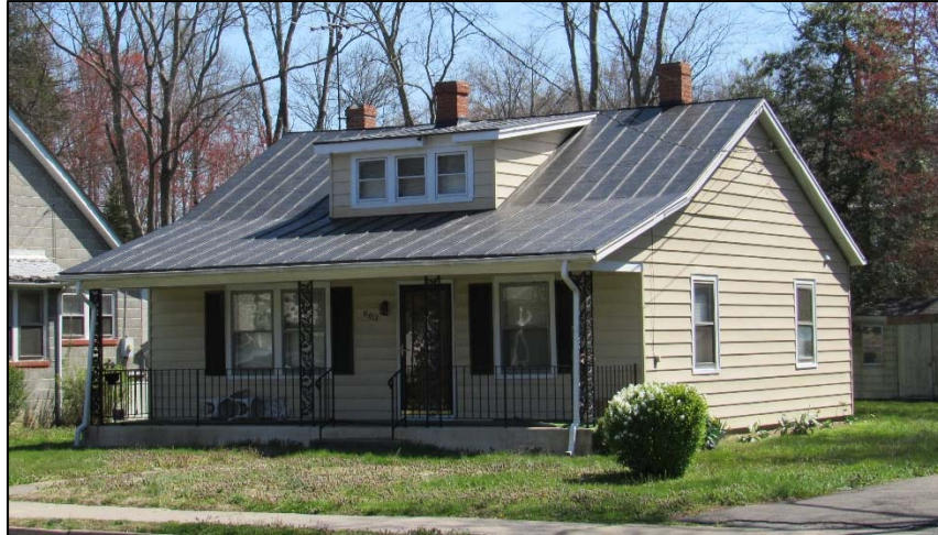
FIGURE 3-89: 603 HENRY STREET, SOUTHWEST OBLIQUE
