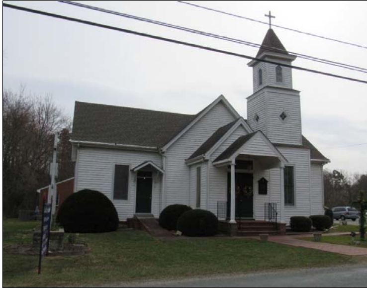
FIGURE 3-154: KENWOOD METHODIST CHURCH (042-0337), WEST ELEVATION
