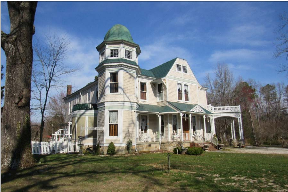
FIGURE 3-123: SOUTHEAST OBLIQUE OF THE CHARLES GWATHMEY HOUSE
