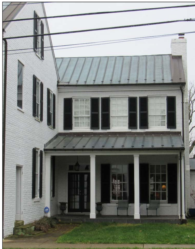
FIGURE 3-16: CIRCA-1990 ADDITION, NORTHEAST ELEVATION
