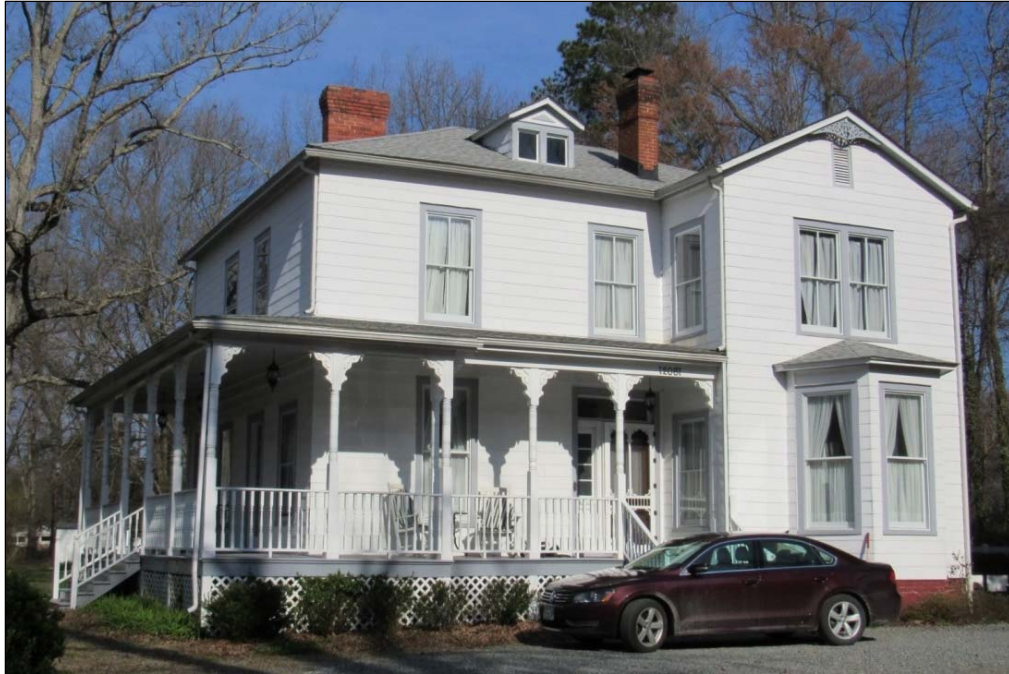
FIGURE 3-132: VIEW OF EAST ELEVATION
