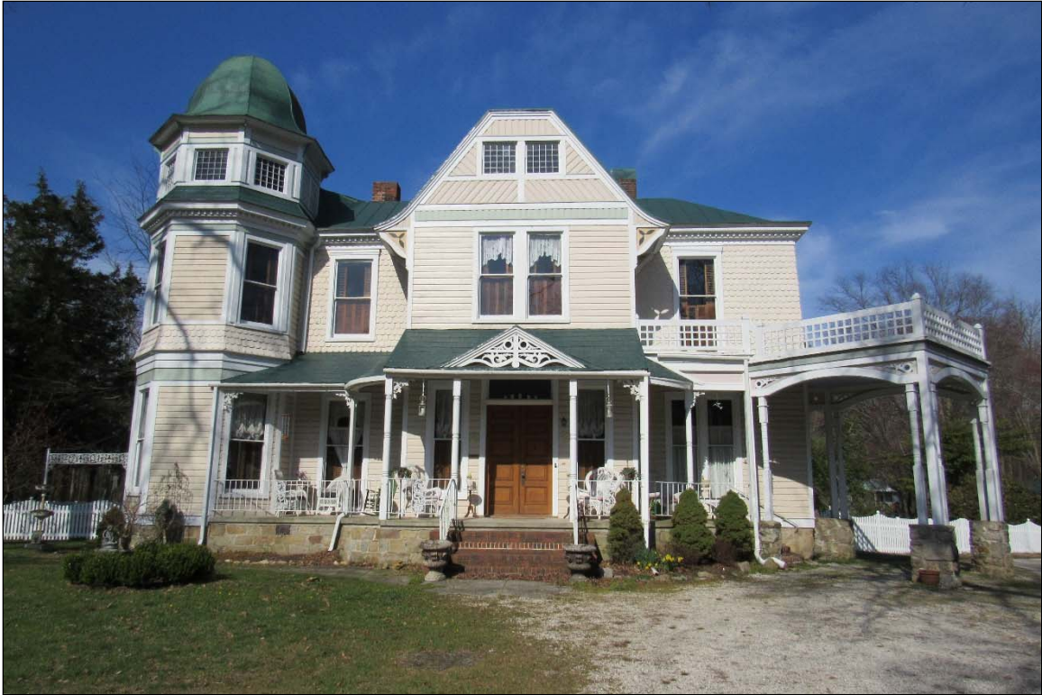
FIGURE 3-122: EAST ELEVATION OF THE CHARLES GWATHMEY HOUSE
