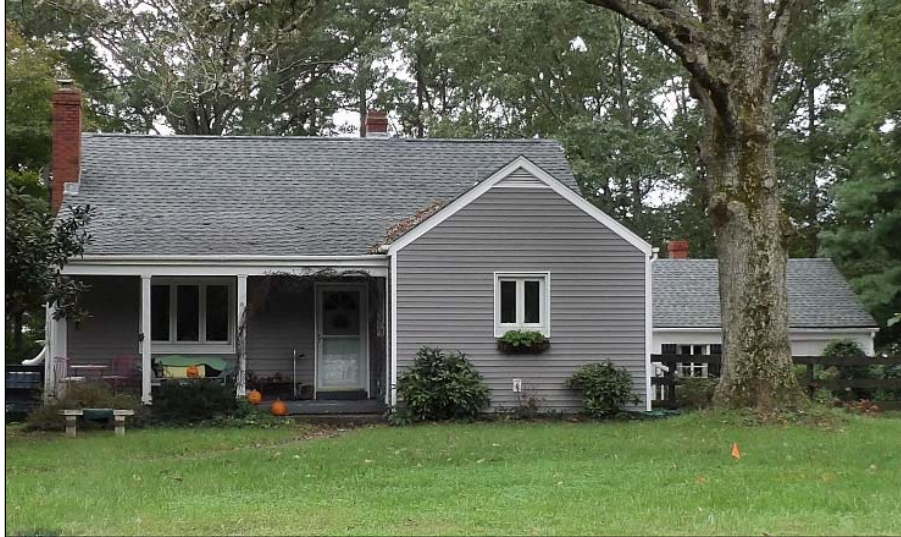
FIGURE 3-166: HOUSE AT 11723 MILL ROAD, NORTH ELEVATION
