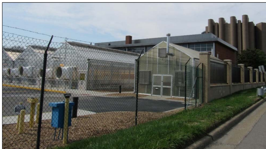
FIGURE 3-216: GREENHOUSES, LOOKING NORTHWEST
