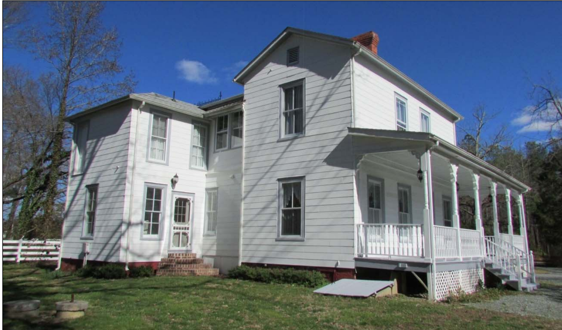
FIGURE 3-136: VIEW OF SOUTHWEST OBLIQUE SHOWING KITCHEN ADDITION AT LEFT
