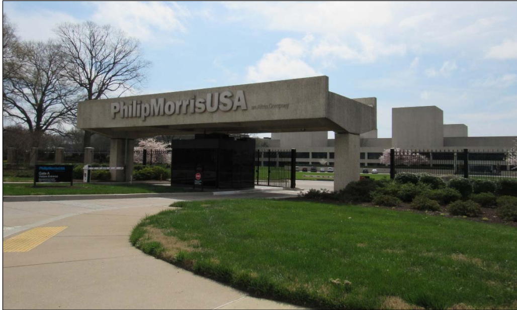
FIGURE 3-218: ENTRY GATE 3, LOOKING SOUTHWEST
