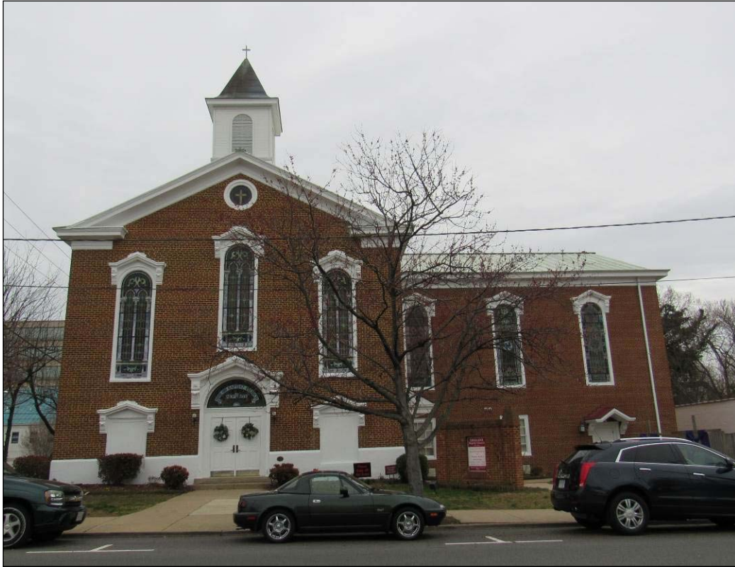
FIGURE 3-43: SHILOH BAPTIST CHURCH (NEW SITE), SOUTHWEST ELEVATION
