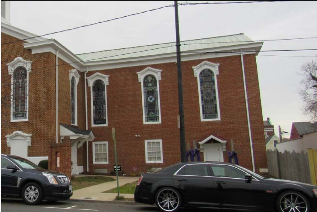
FIGURE 3-46: CIRCA-1980 ADDITION, SOUTHWEST ELEVATION
