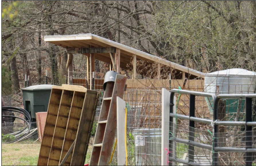
FIGURE 3-78: CIRCA-2017 ANIMAL SHELTER, LOOKING SOUTHWEST
