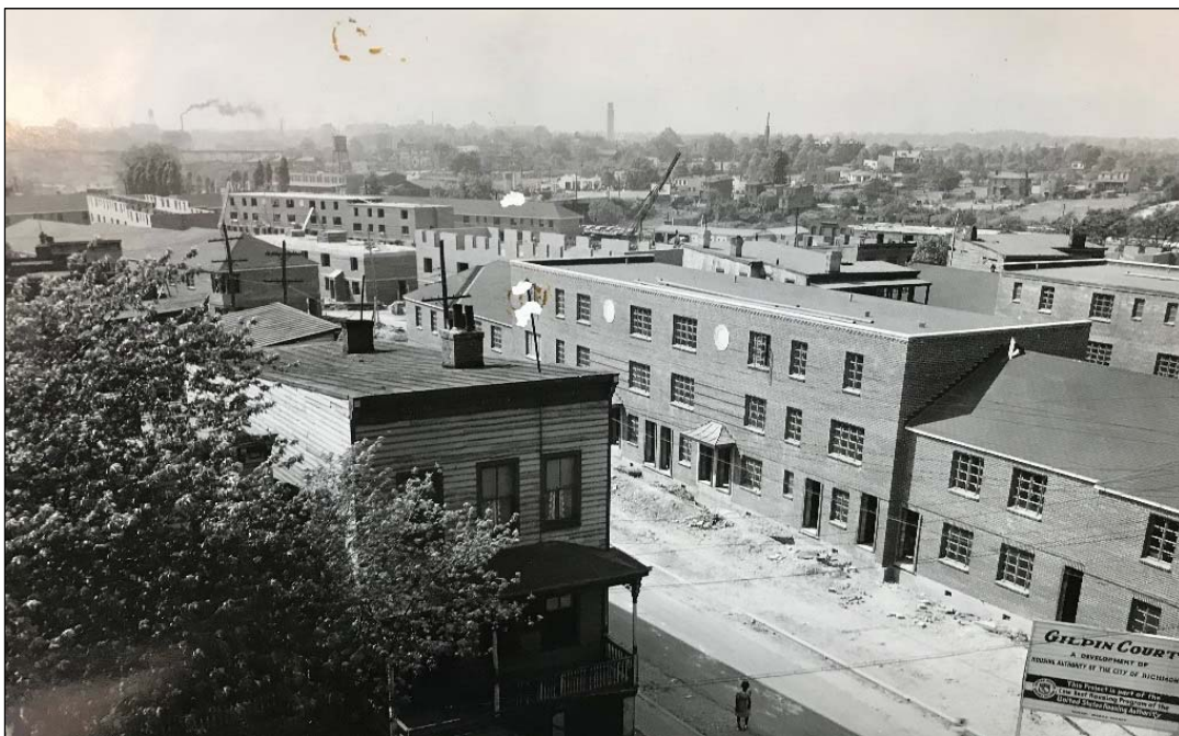
FIGURE 3-187: GILPIN COURT APARTMENT COMPLEX IN THE MIDST OF CONSTRUCTION IN 1942 (RRHA 1942)
