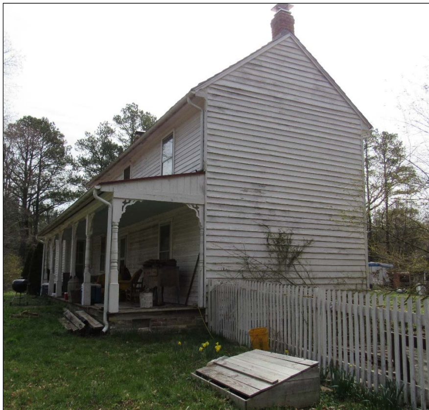
FIGURE 3-74: DWELLING AT DRY BRIDGE, WEST ELEVATION
