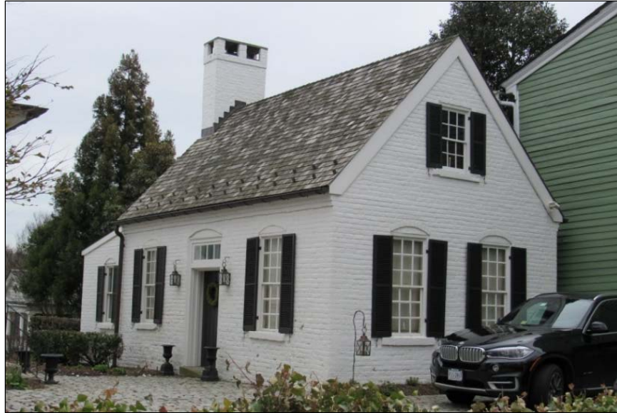
FIGURE 3-35: NORTHWEST OBLIQUE VIEW OF KITCHEN
