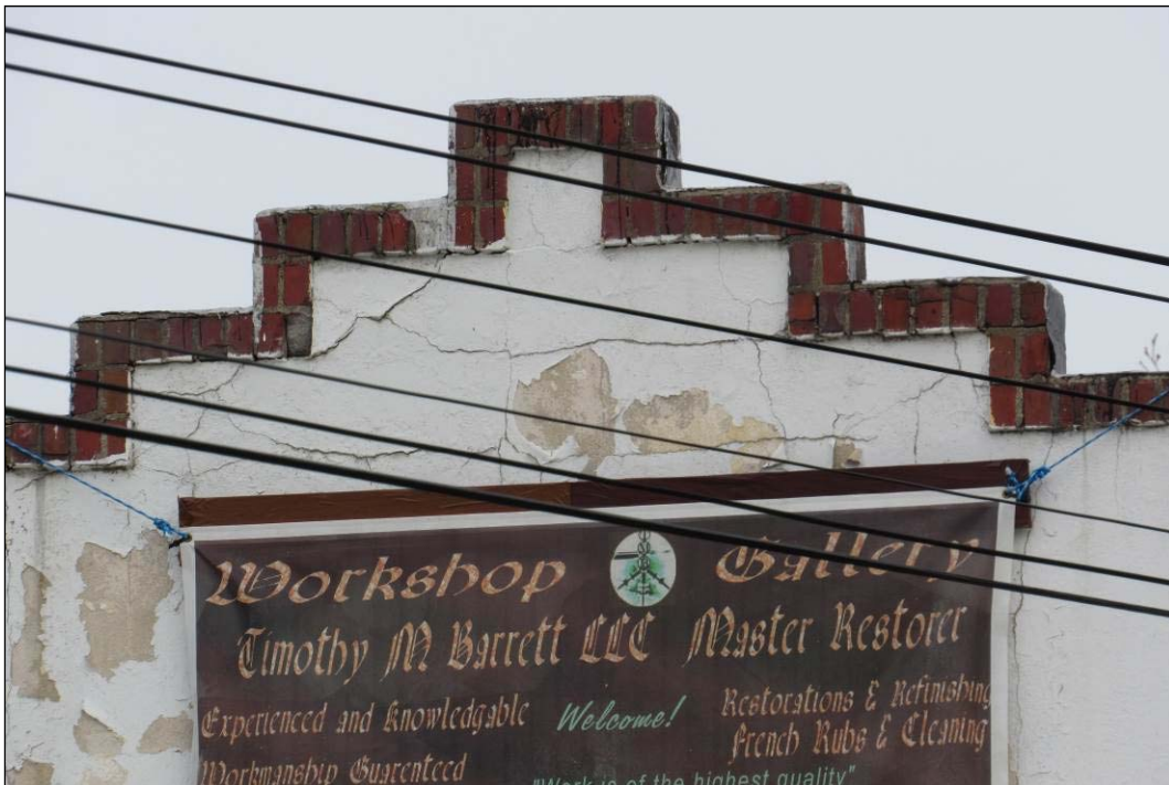
FIGURE 3-178: PARAPET DETAIL ON FAÇADE, FACING NORTH
