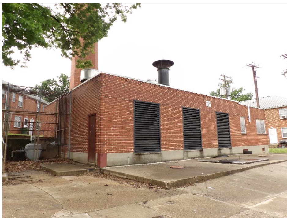
FIGURE 3-195: GILPIN COURT APARTMENT COMPLEX, CENTRAL HEATING PLANT, LOOKING SOUTH
