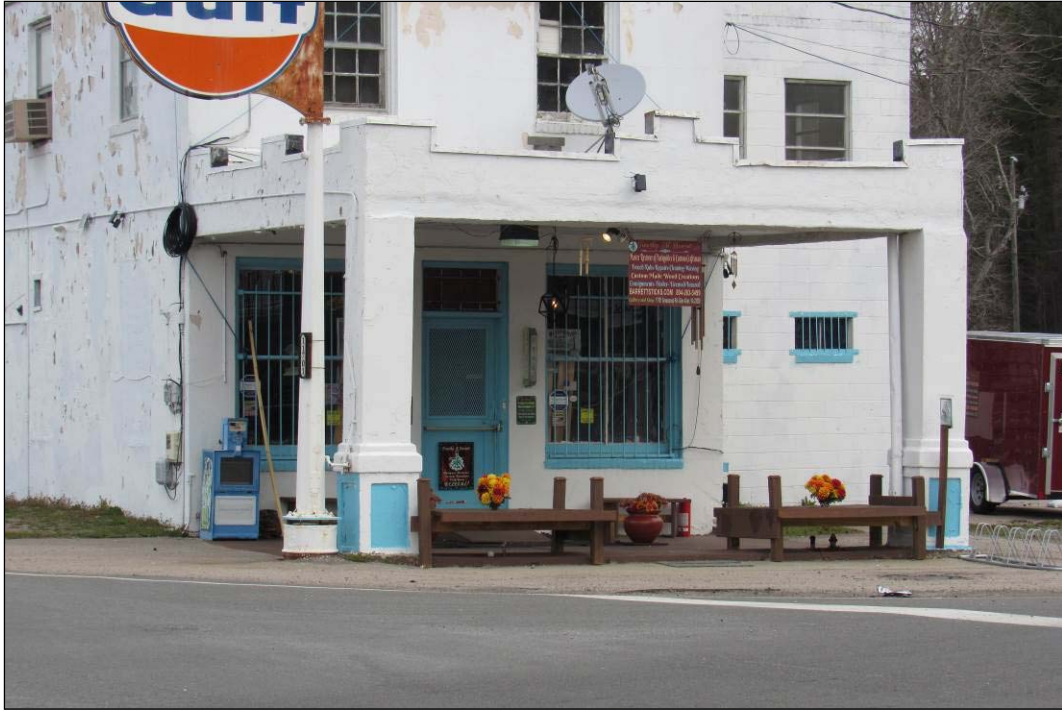
FIGURE 3-179: CANOPY DETAIL, FACING NORTH
