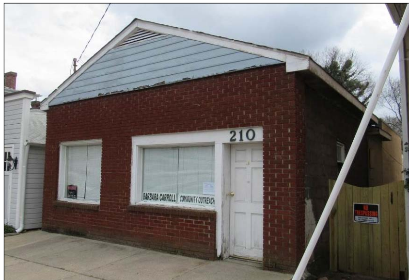
FIGURE 3-54: CIRCA-1940 COMMERCIAL OUTBUILDING, WEST OBLIQUE
