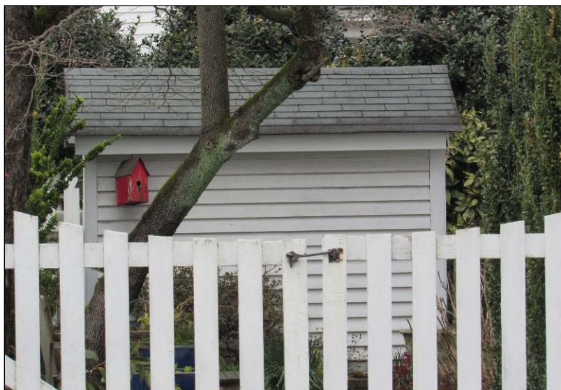
FIGURE 3-17: SHED, SOUTH ELEVATION
