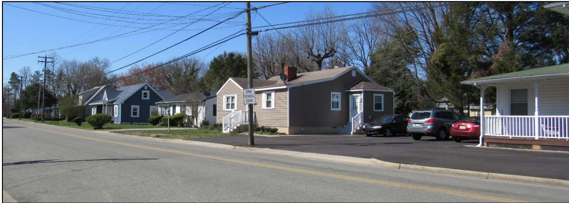
FIGURE 3-92: VIEW ALONG HENRY STREET, LOOKING SOUTH
