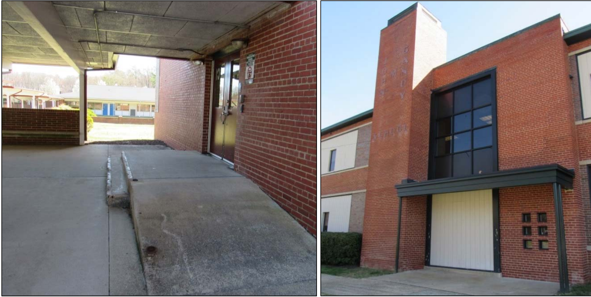
FIGURE 3-117: ELEMENTARY SCHOOL CONNECTION (LEFT) AND FORMER ENTRY BAY (RIGHT)
