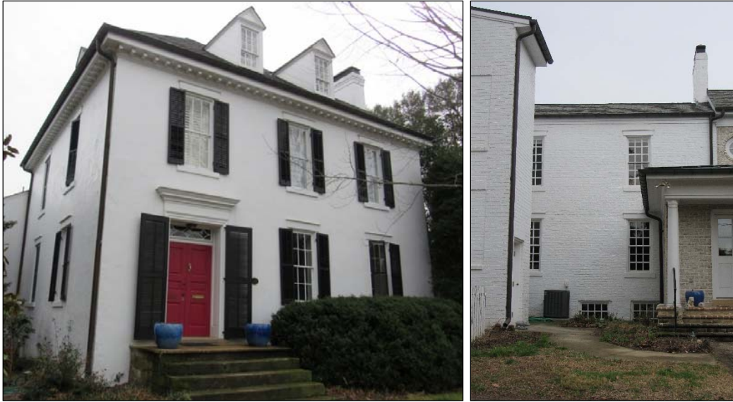
FIGURE 3-24: NORTHWEST OBLIQUE (LEFT) AND SOUTHEAST ELEVATION DETAIL (RIGHT)
