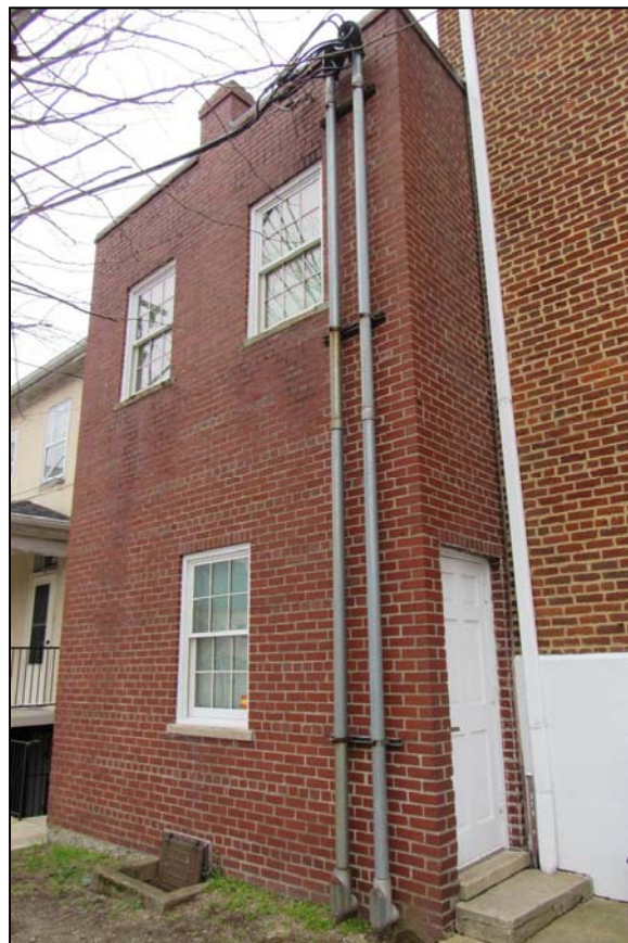
FIGURE 3-47: CIRCA-1960 ADDITION, NORTHWEST ELEVATION
