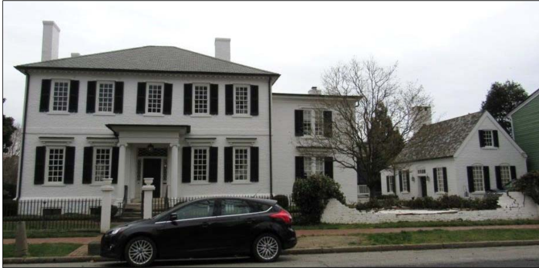
FIGURE 3-32: SOUTHWEST ELEVATION WITH KITCHEN
