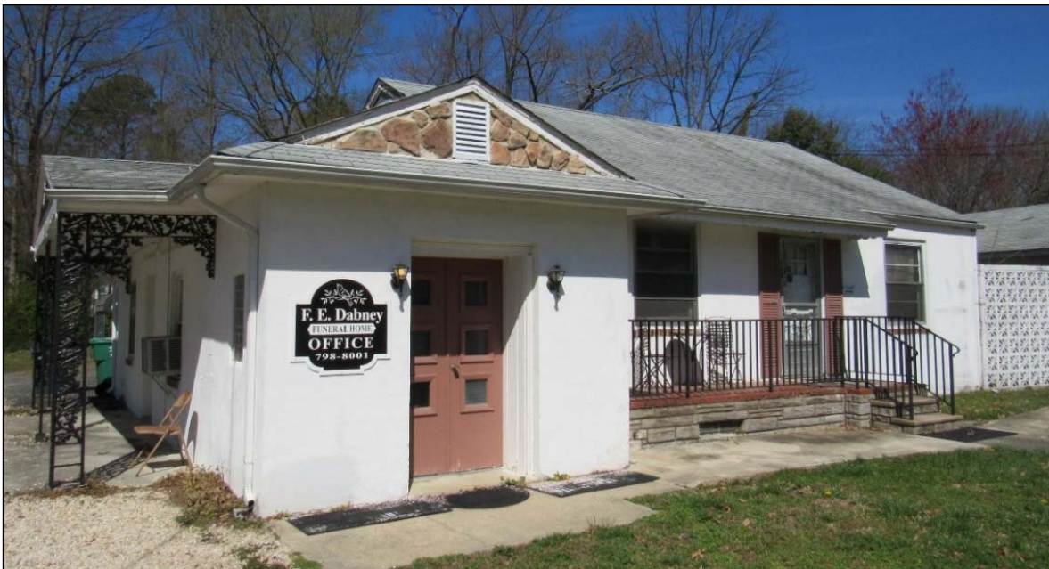
FIGURE 3-103: OFFICE ADDITION, SOUTH OBLIQUE
