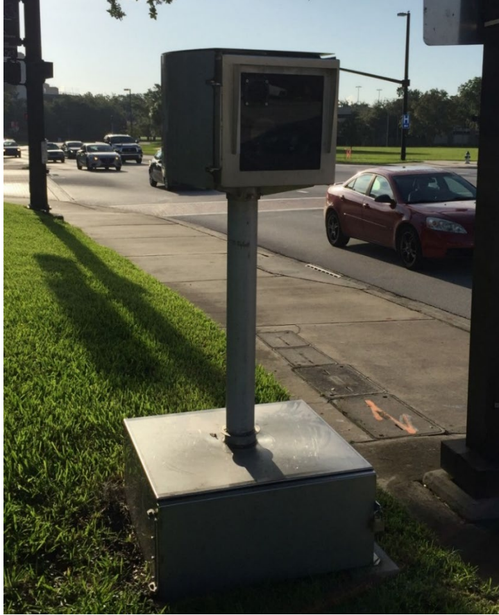
Figure 7. Photo Enforcement System at East Princeton Street
