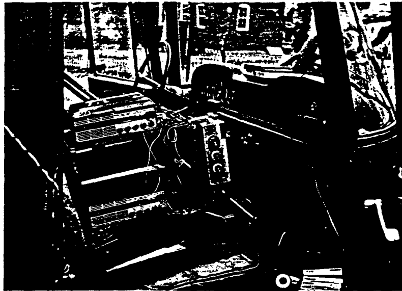
Figure 31. Electronics Inside Truck Cab
