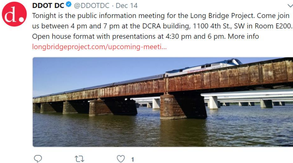
Figure 3-1 | DDOT Tweet on the Long Bridge Public Information Meeting, December 14, 2017
