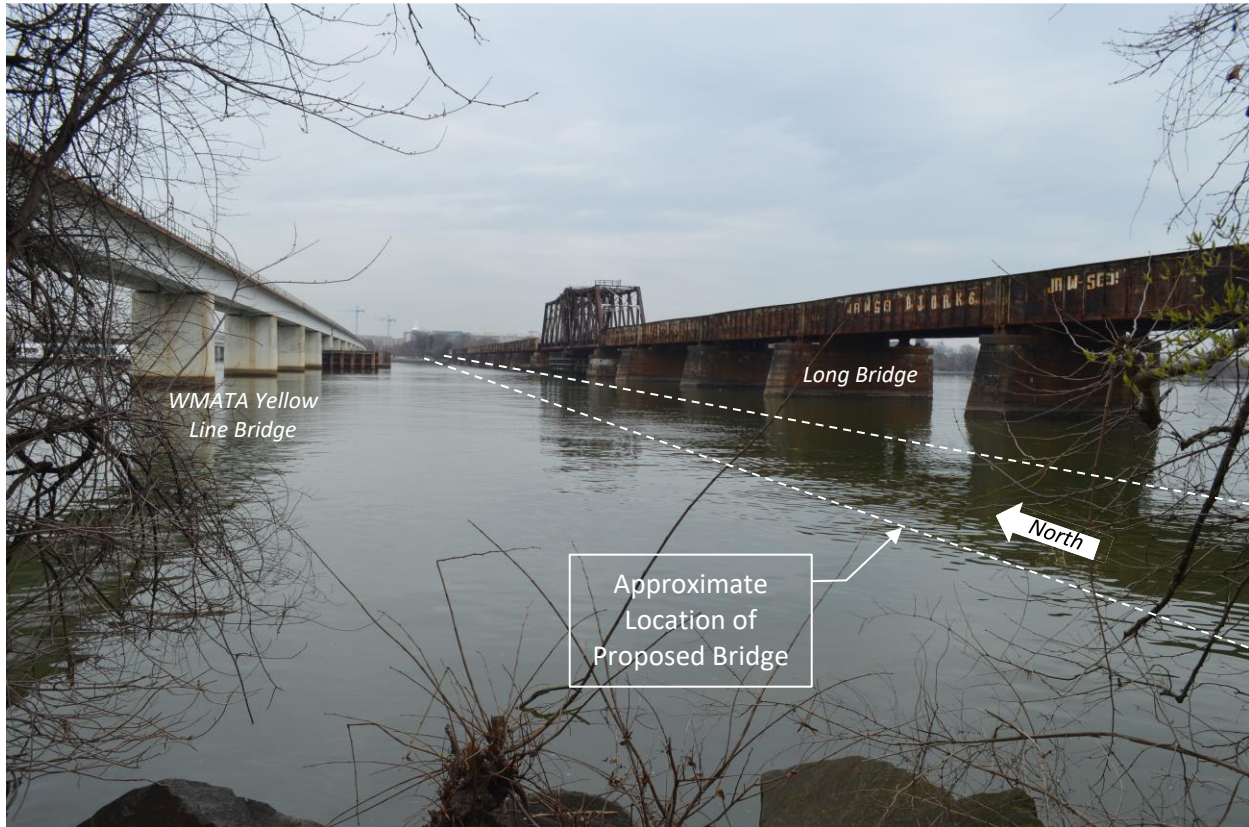
Figure 3-1 | Approximate Location of Proposed Upstream Bridge (looking north)
