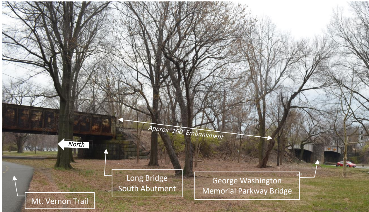
Figure 2-7 | Track Embankment beyond South Abutment
