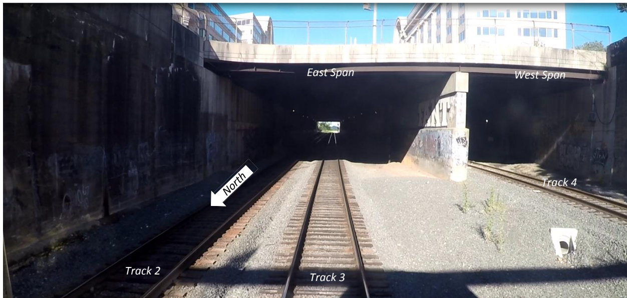
Figure 2-4 | 12 th Street SW Looking South
