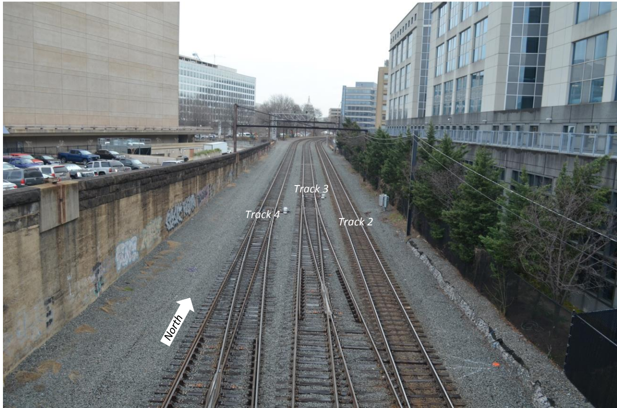
Figure 2-8 | Retaining Walls Looking North from L'Enfant Plaza
