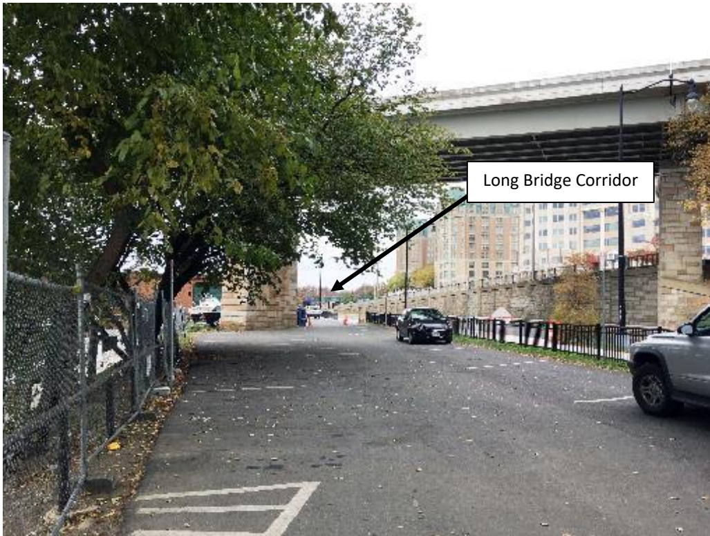
Figure 12-18 | View 17: DC Marina Looking North along Maine Avenue SW to Long Bridge Corridor
