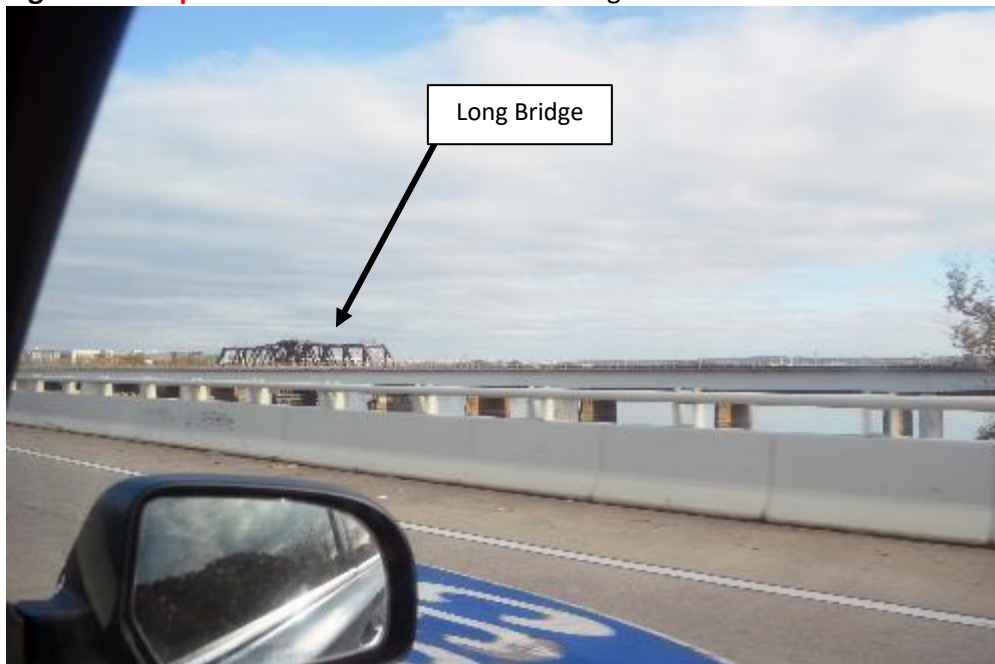
Figure 12-13 | View 12: I-395 Northbound Looking Southeast
