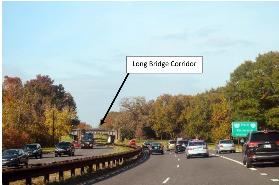
Figure 12-9 | View 8: George Washington Memorial Parkway Looking North to Long Bridge Corridor
