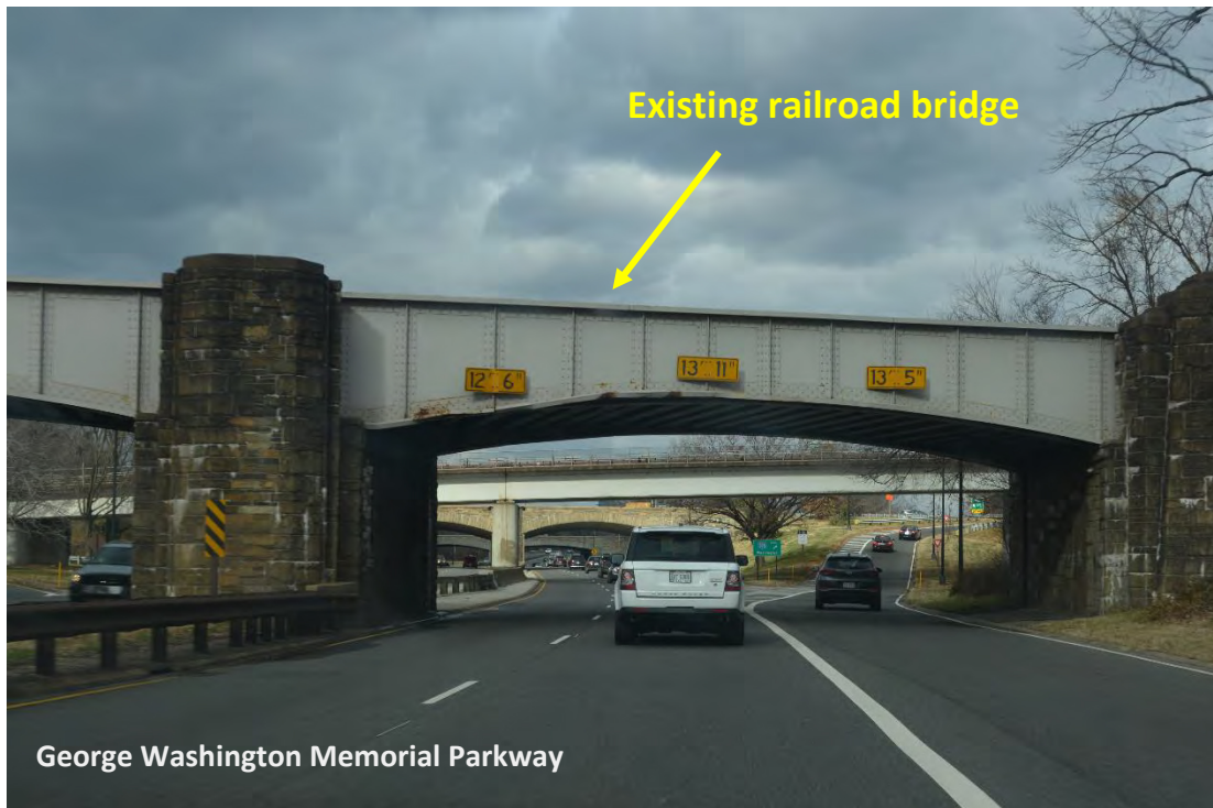
View D, Existing Conditions
