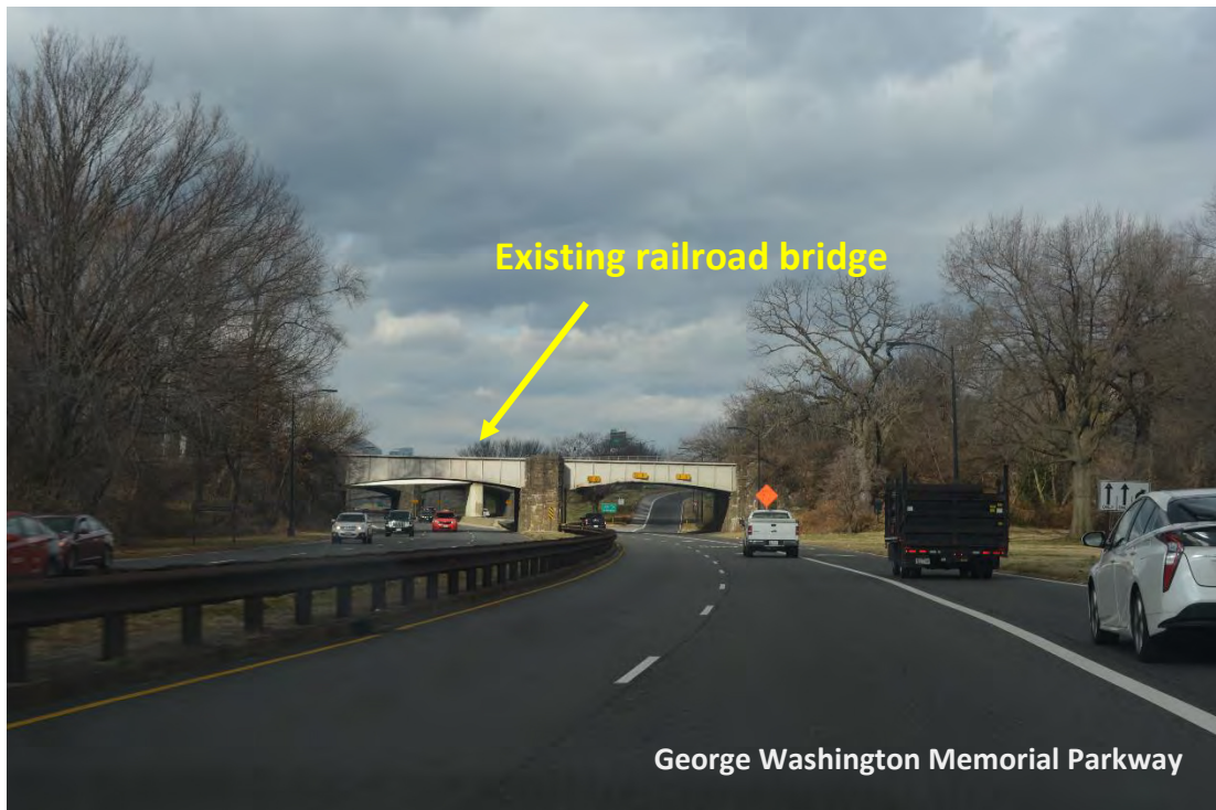
View E, Existing Conditions
