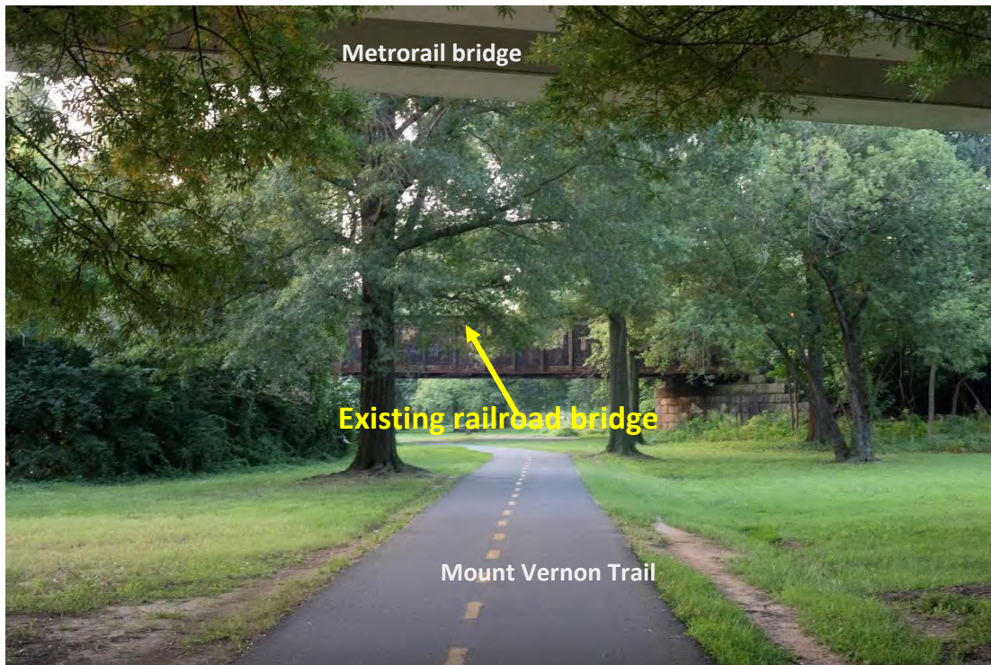
View G, Existing Conditions
