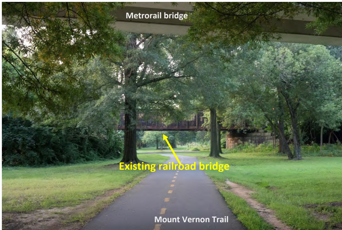
View G, Existing Conditions
