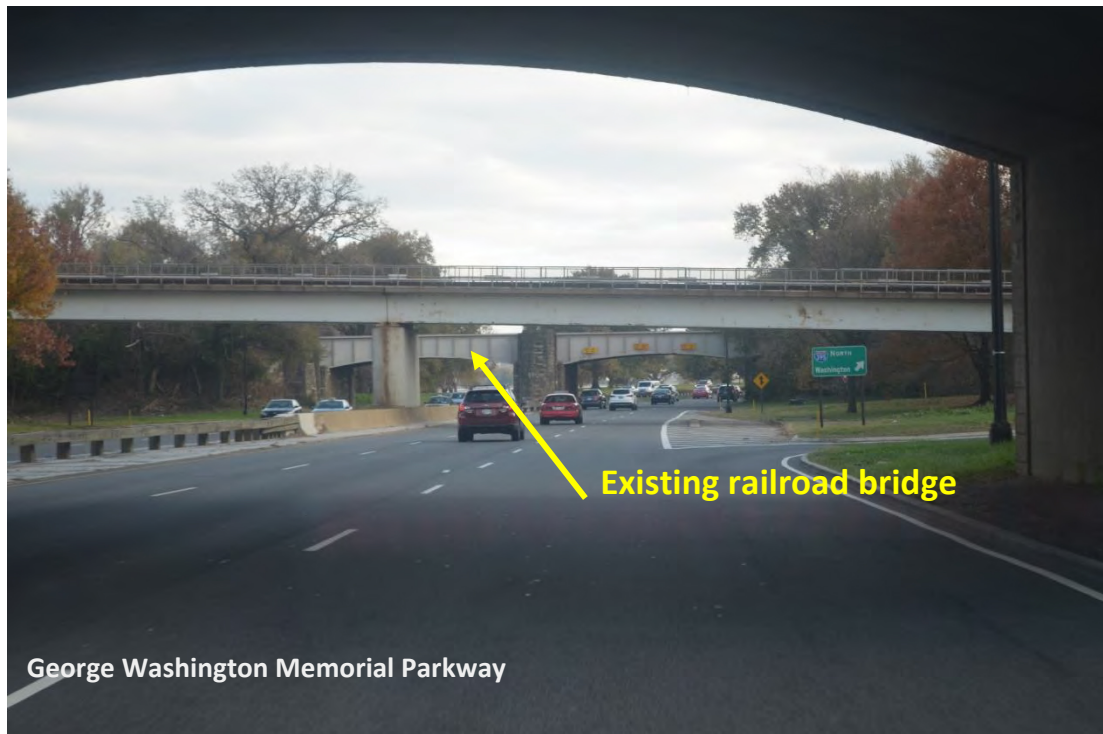
View C, Existing Conditions
