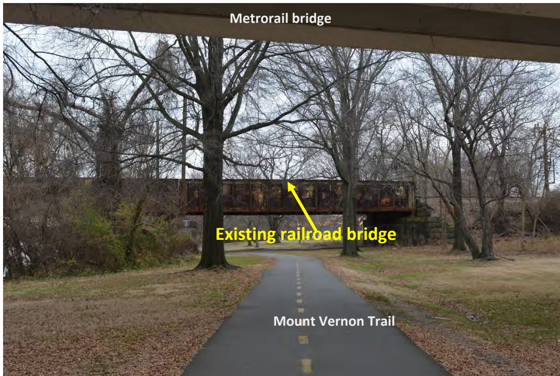
View G, Existing Conditions
