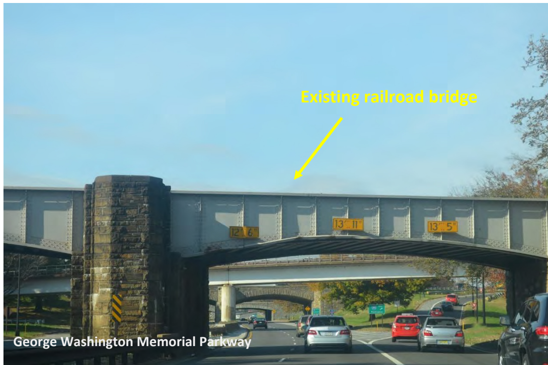
View D, Existing Conditions
