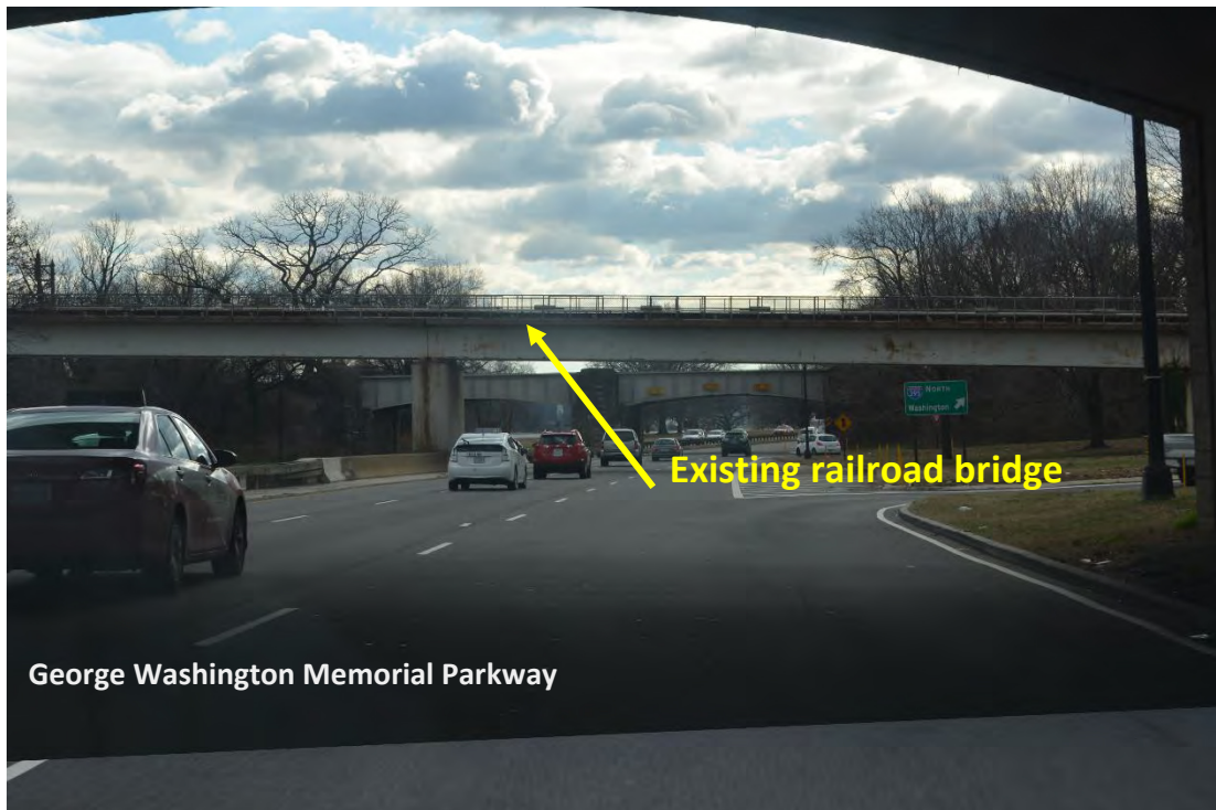
View C, Existing Conditions
