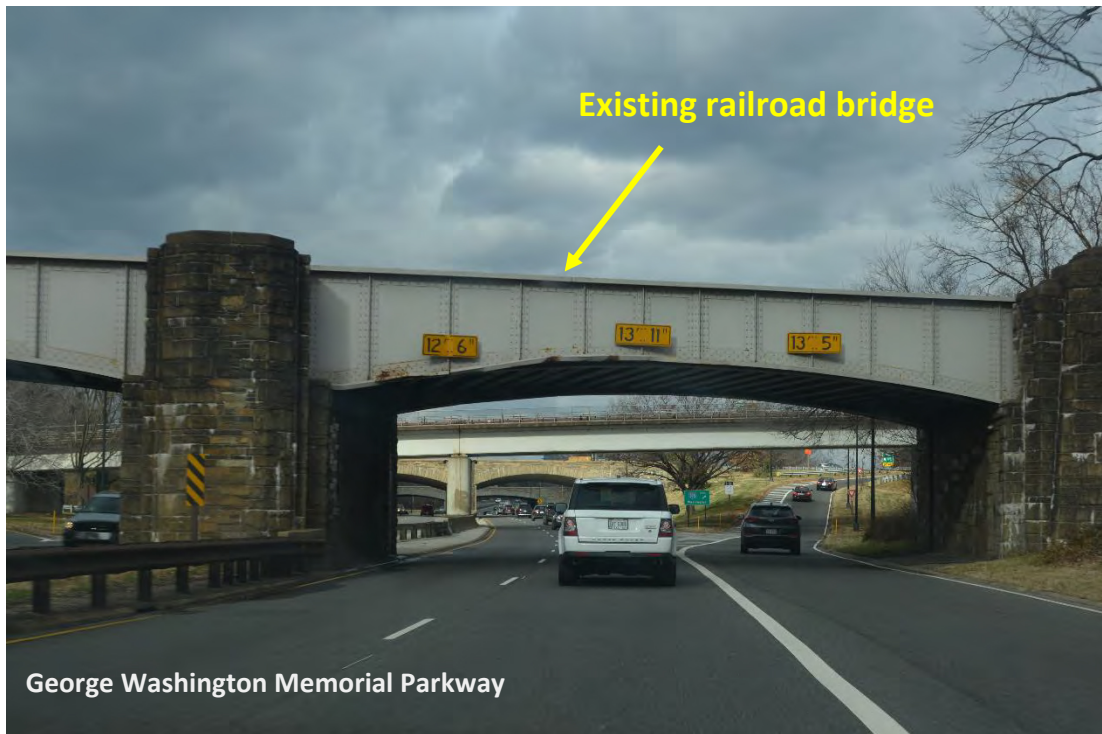
View D, Existing Conditions
