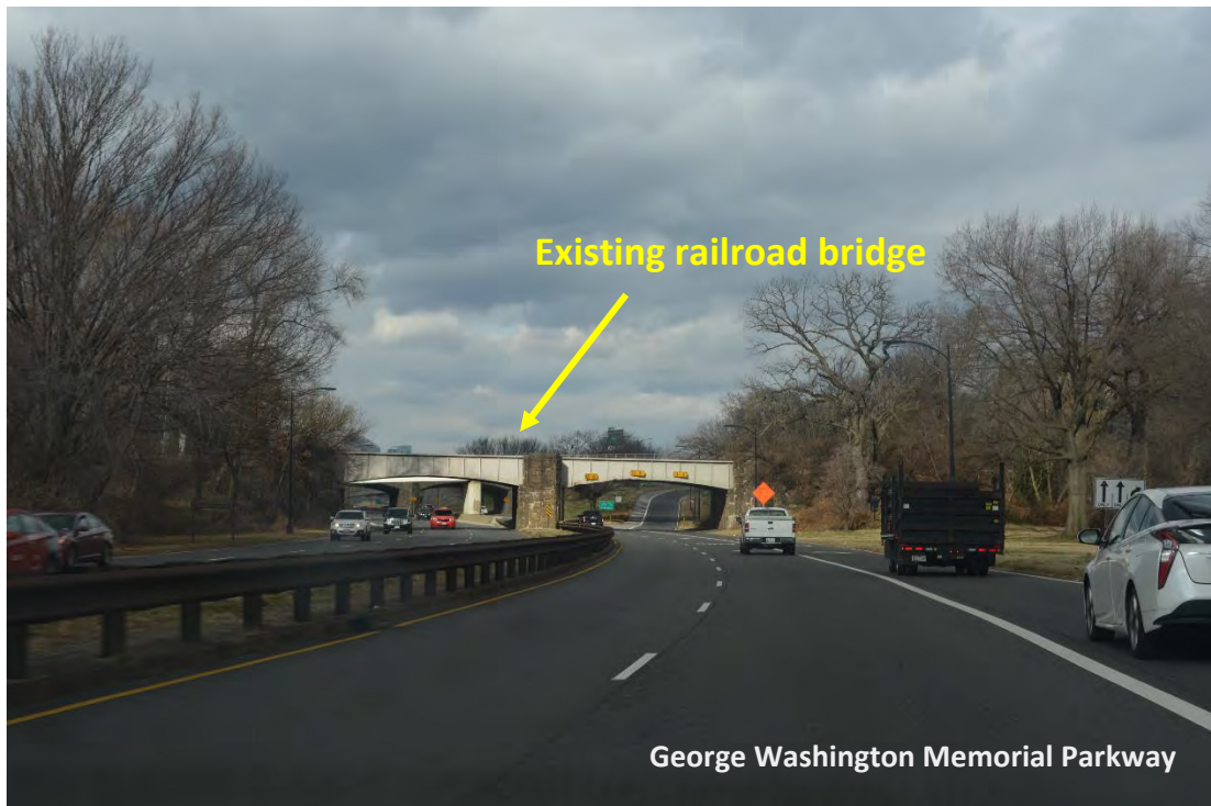
View E, Existing Conditions
