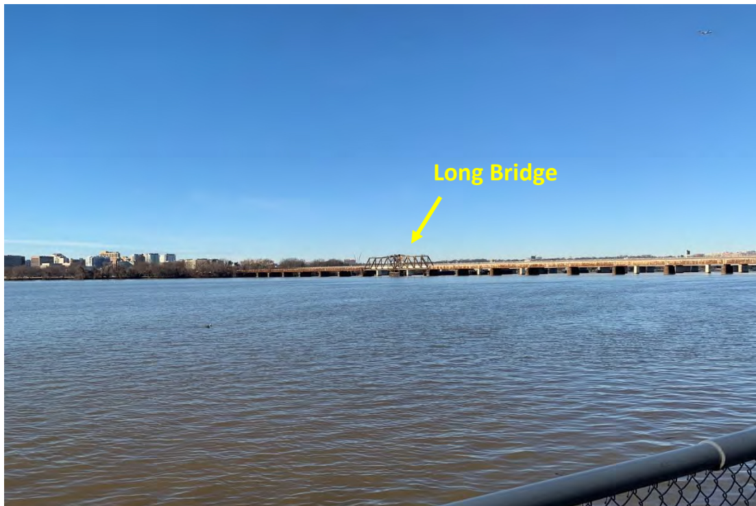
View L, Existing Conditions
