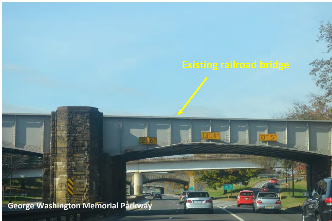
View D, Existing Conditions
