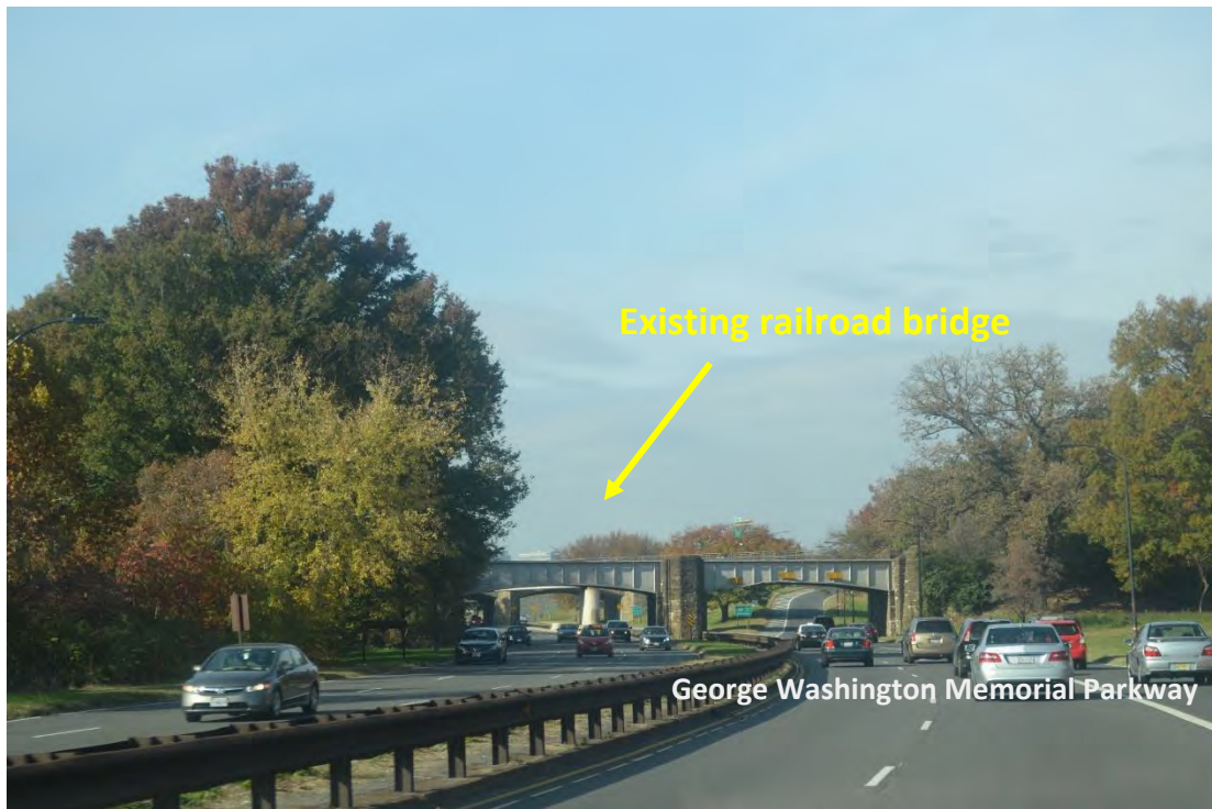
View E, Existing Conditions
