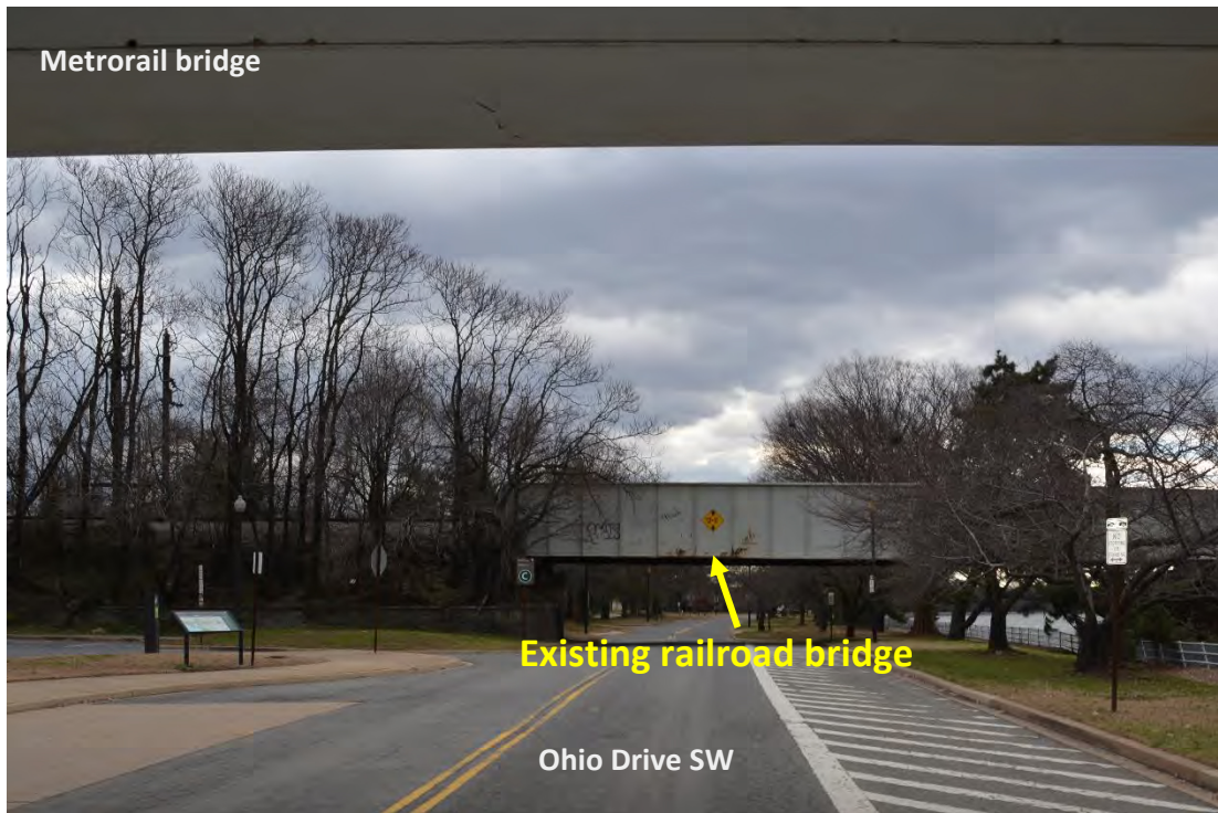
View J, Existing Conditions
