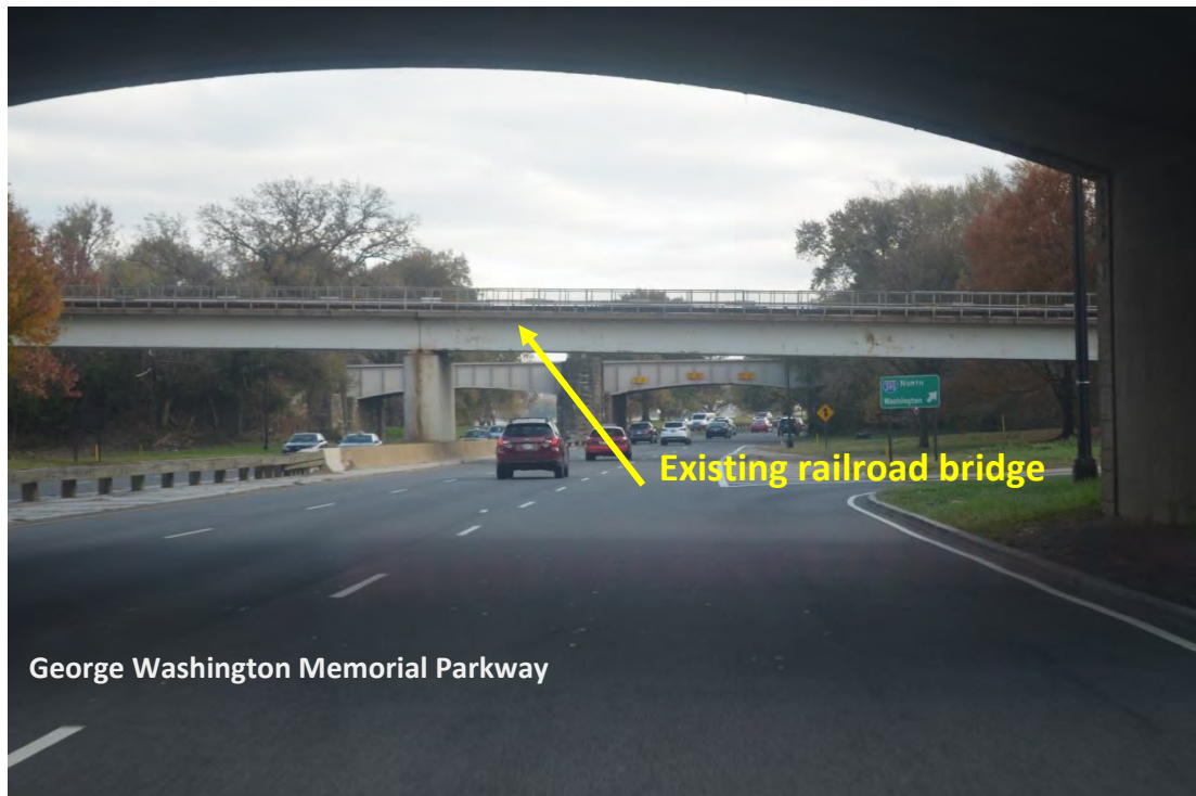
View C, Existing Conditions
