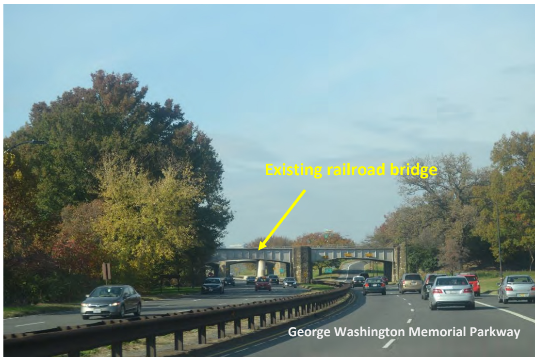
View E, Existing Conditions
