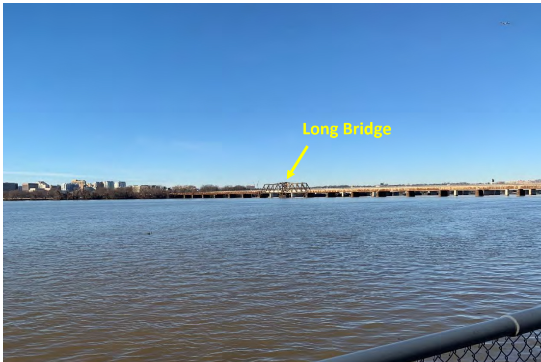
View L, Existing Conditions
