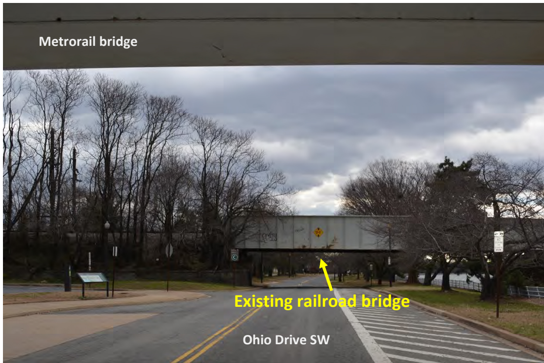
View J, Existing Conditions
