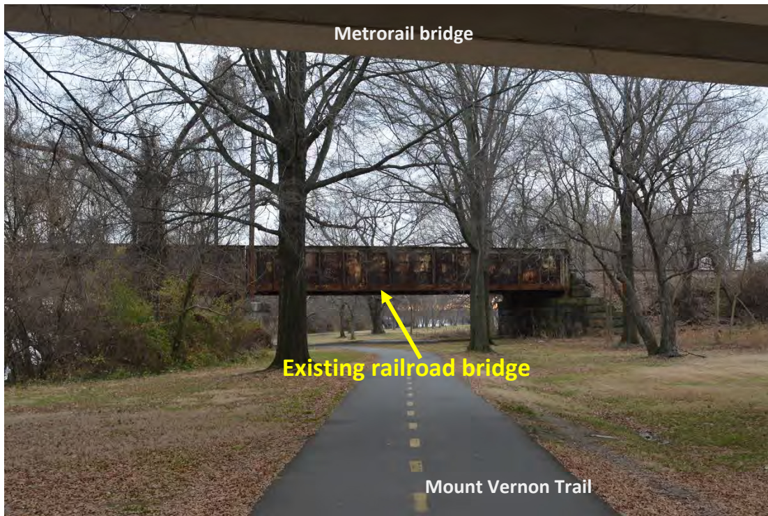
View G, Existing Conditions
