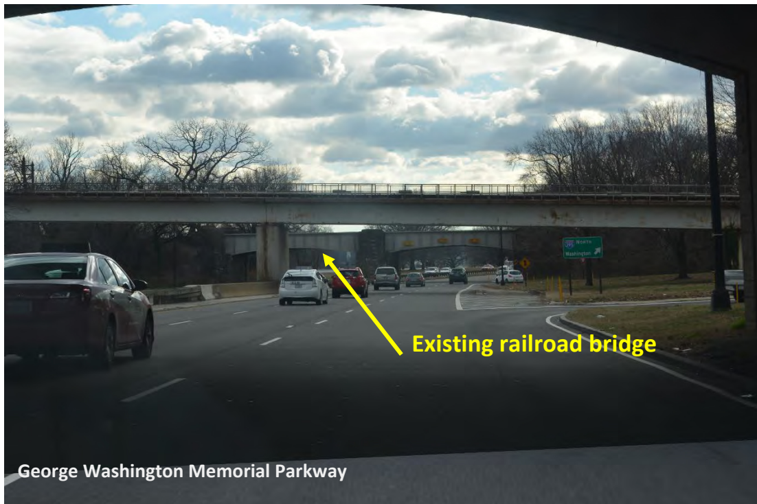
View C, Existing Conditions
