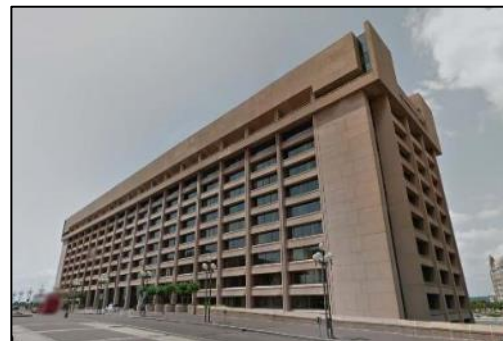
Figure 3-45 | USPS Building (Google Maps)
