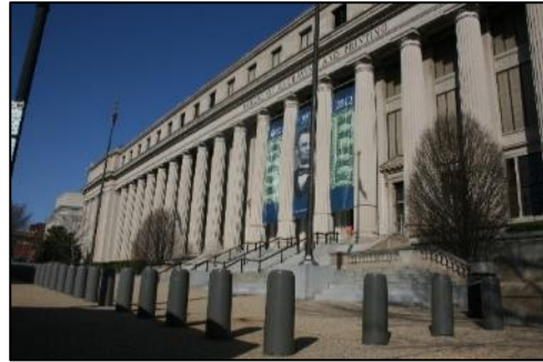
Figure 3-15 | BEP Main Building
