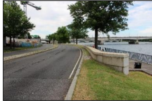
Figure 3-3 | Rock Creek and Potomac Parkway
