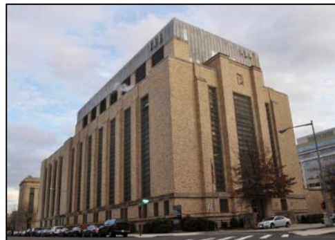
Figure 3-11 | Central Heating Plant
