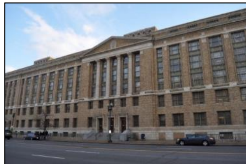
Figure 3-14 | USDA South Building
