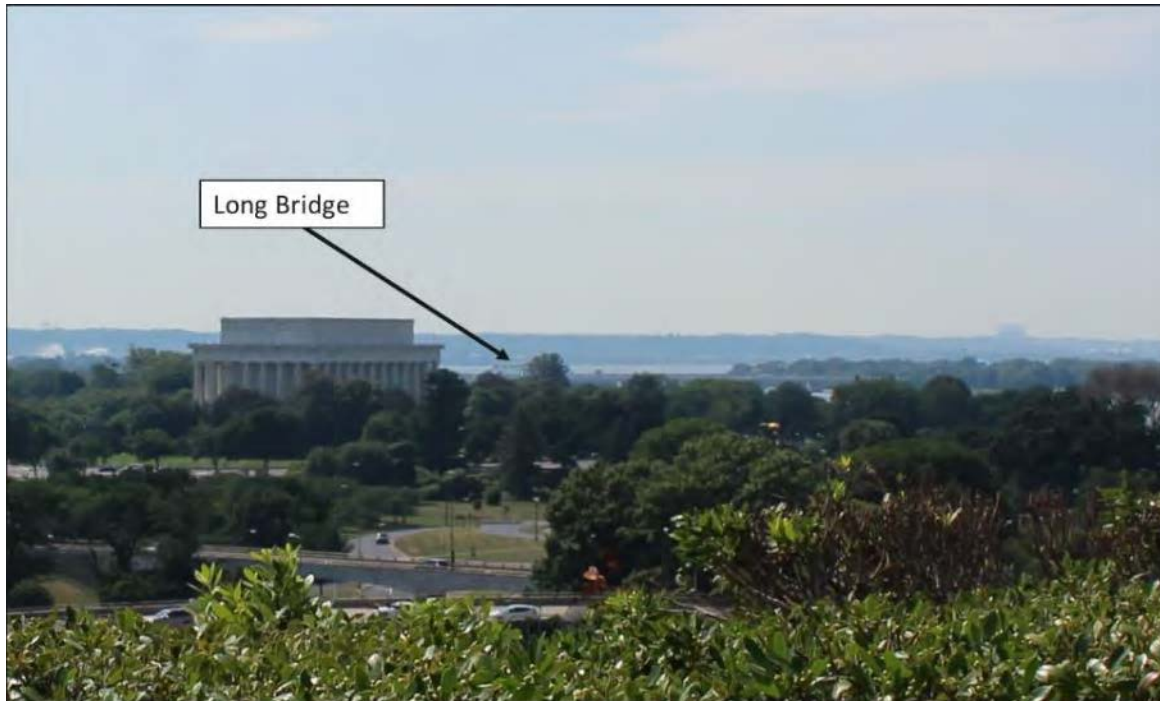
Figure 2-7 | Photograph location 2. Long Bridge from the west section of the Kennedy Center upper terrace, facing southeast
