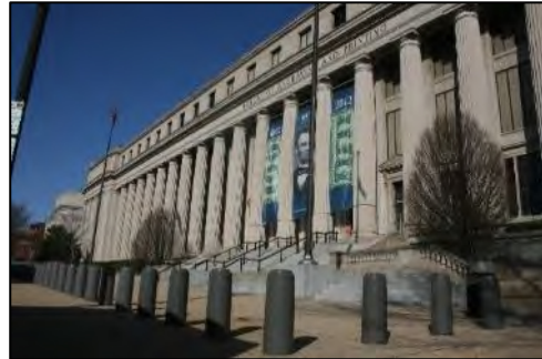
Figure 3-15 | BEP Main Building
