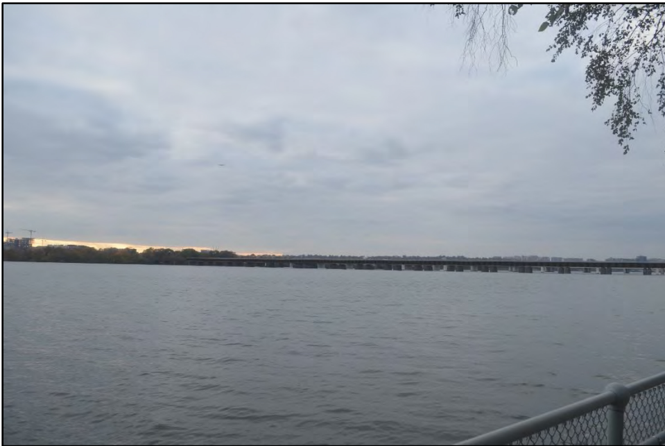
Action Alternative B: New railroad bridge visible.
