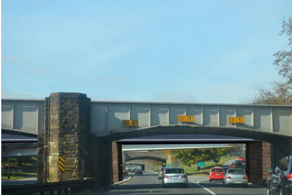
Action Alternative A: New railroad bridge visible behind existing railroad bridge.
