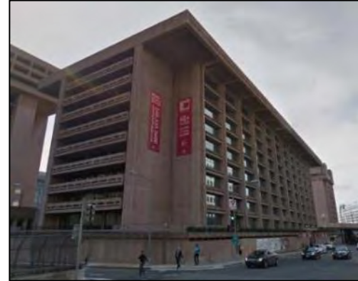
Figure 3-42 | Astral Building (Google Maps)
