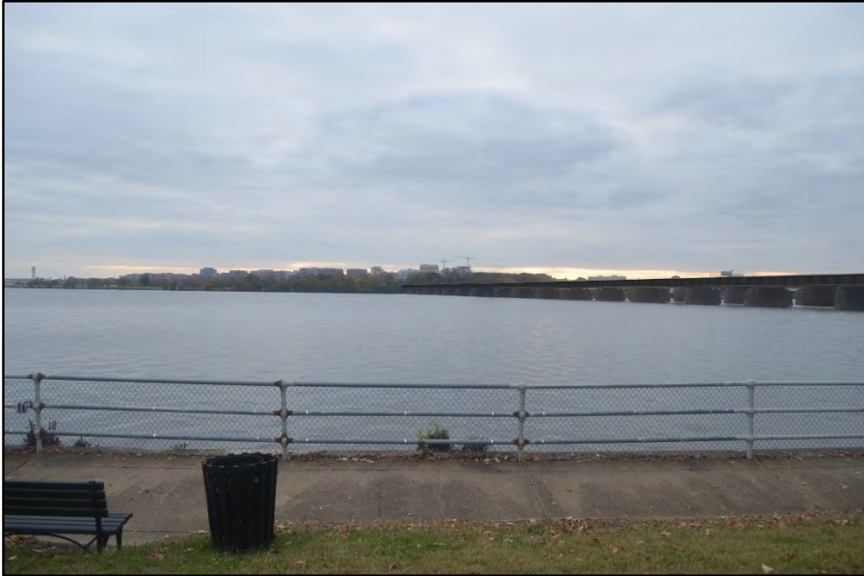
Action Alternative B: New railroad bridge visible.
