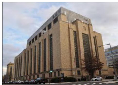
Figure 3-11 | Central Heating Plant
