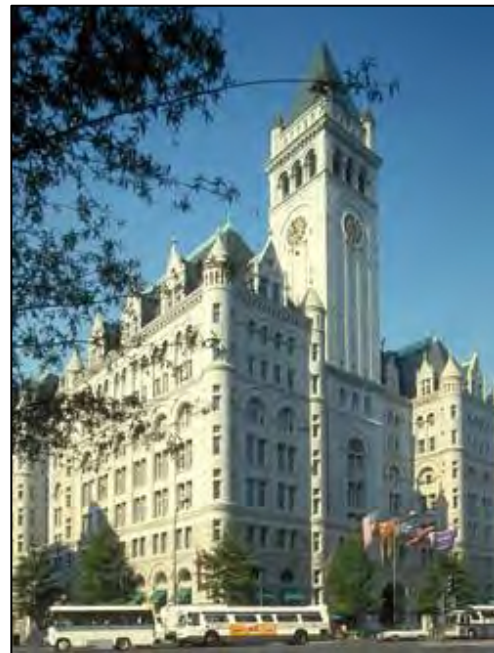
Figure 3-30 | The Old Post Office (National Park Service)
