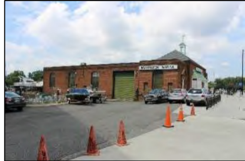
Figure 3-36 | Washington Marina Building
