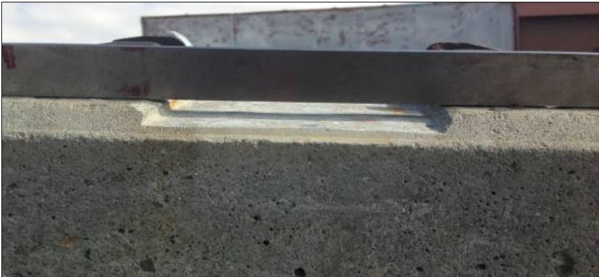
Figure 10. Example Showing Uniform RSD Depth Profile
