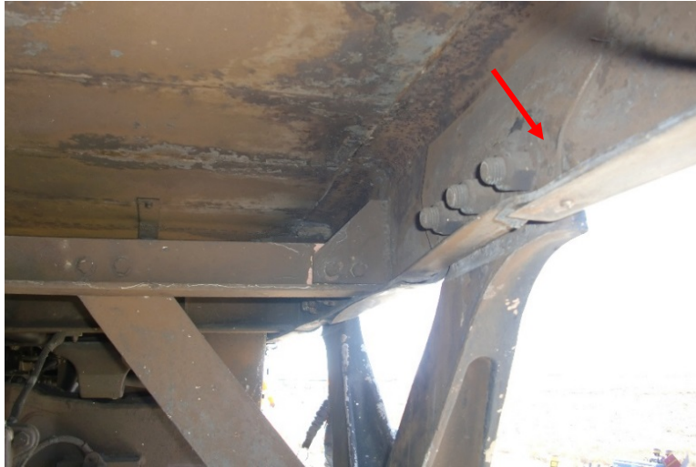
Figure 16. M1 side sill buckled at front-left truck connection (interior view)
