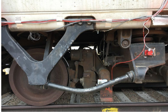
Figure 44. M1 front-left traction rod deformed more after 8 mph test
