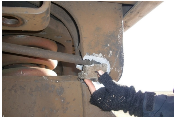
Figure 17. M1 side sill front-left truck connection damage
