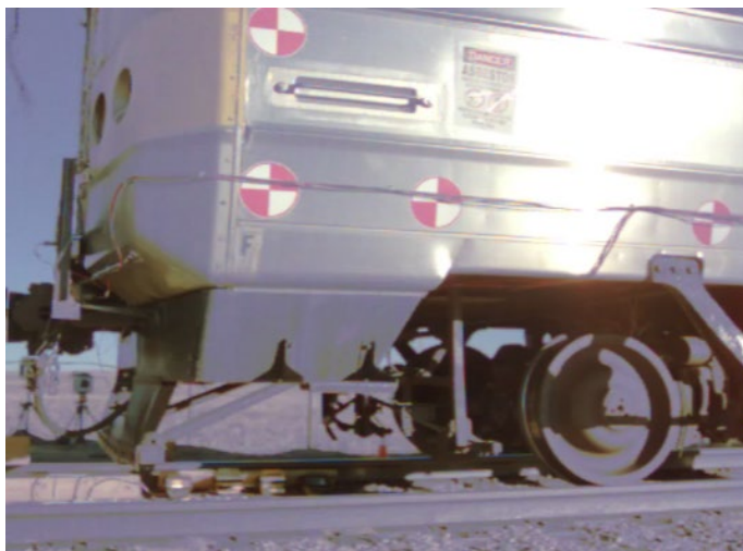
Figure 63. Conventional coupling test: Dimpling of M1 shell at front left side sill truck connection after 5.7 mph impact test
