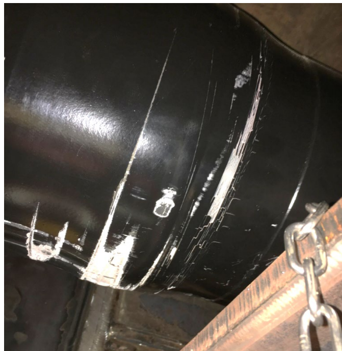
Figure 49. Cracked paint on the left side of the PBC deformation tube, indicating tube crush
