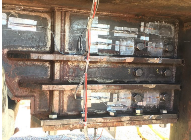
Figure 35. Exterior view of the shear bolts installed through the draft pocket
