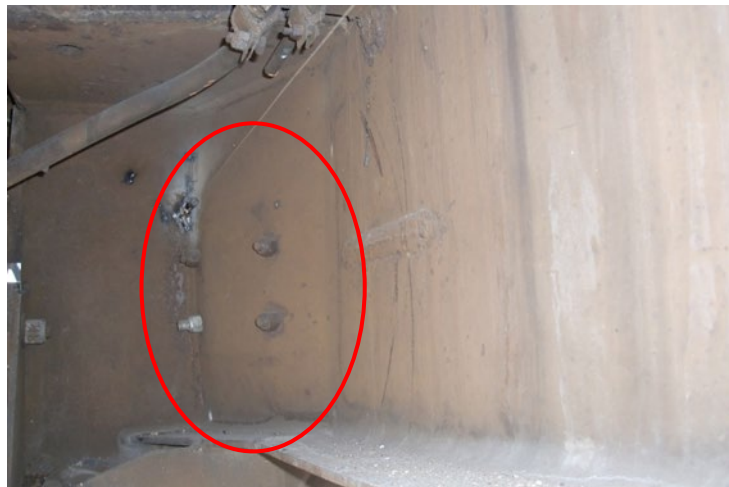
Figure 11. Bulging of M1 left draft sill due to coupler shank pushing on coupler stops inside bellmouth
