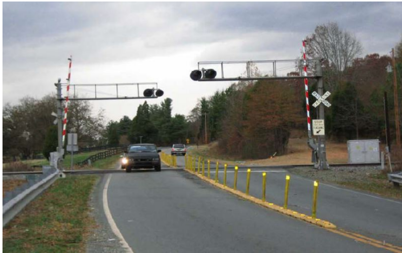
Figure 3.7 An upgraded grade-crossing with four-quadrant gates, train approaching warning devices, and traffic channelization devices (Bien-Aime, 2009)
