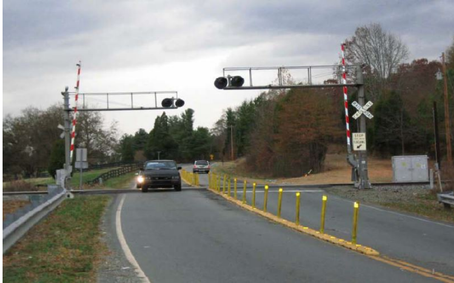
Figure C-7: An Upgraded Grade Crossing with Four-Quadrant Gates, Train Approaching Warning Devices, and Traffic Channelization Devices (Bien-Aime, 2009)
