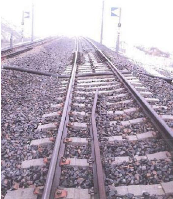
Figure C-4: Guard Rail Protection (Abtahi, 2013)
