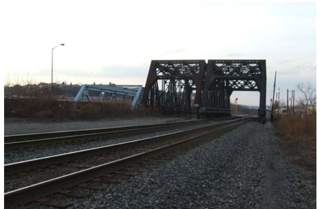
Chartiers Creek Bridge Modification
