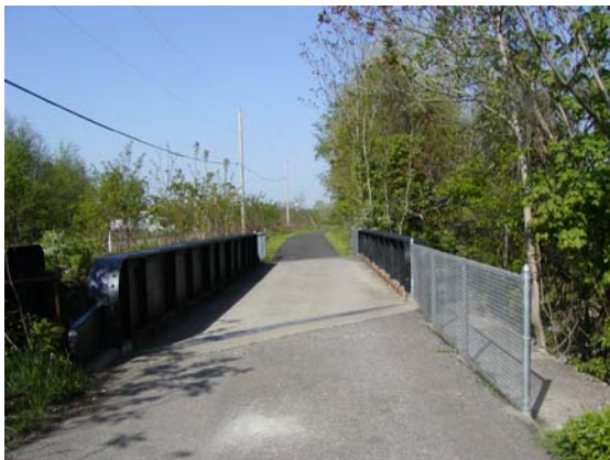
Kent Hike and Bike Trail Bridge Raising
