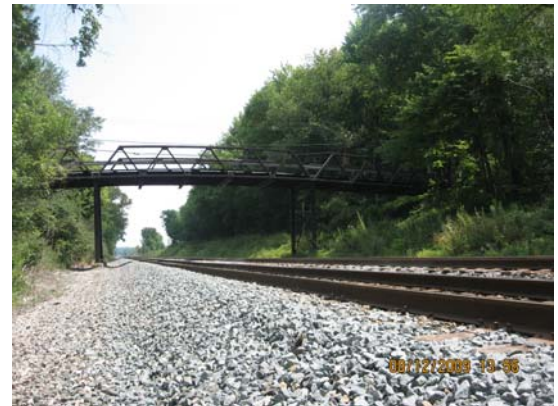
Fifth Street Bridge, Eligible to the NRHP
