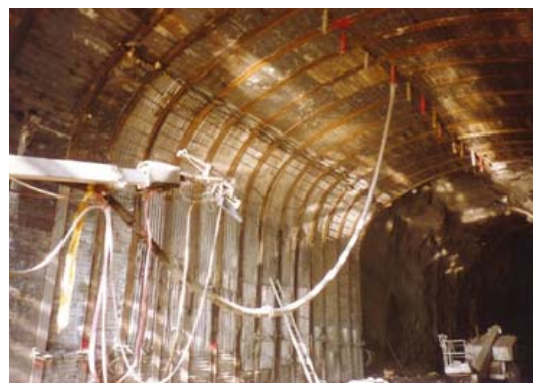
Total Arch Liner Replacement
