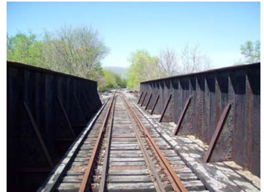
Mexico Farms Railroad Bridge Removal
