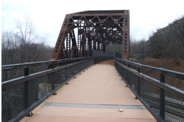
Blue Lick Truss Trail Entrance
