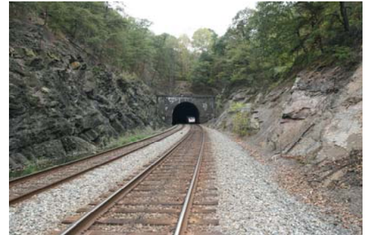
Stuart Tunnel East Portal
