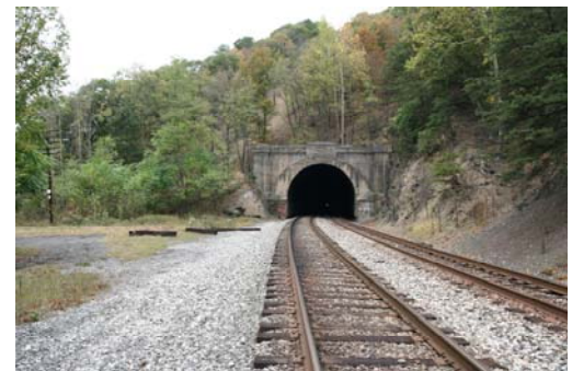
Randolph Tunnel West Portal
