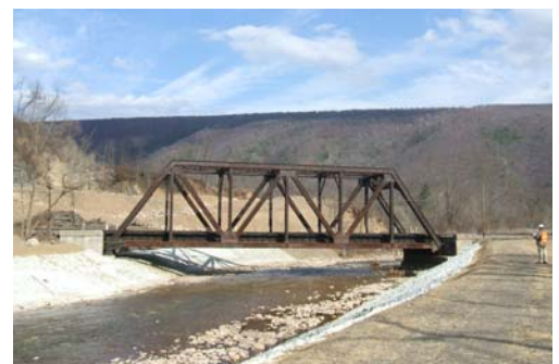
Hyndman Railroad Bridge Modification
