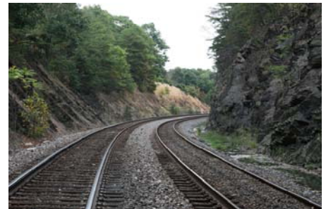
Stuart Tunnel View from East Portal
