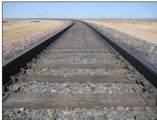
Figure 1. Southern Yellow Pine Crosstie Test Zone Installed at FAST
