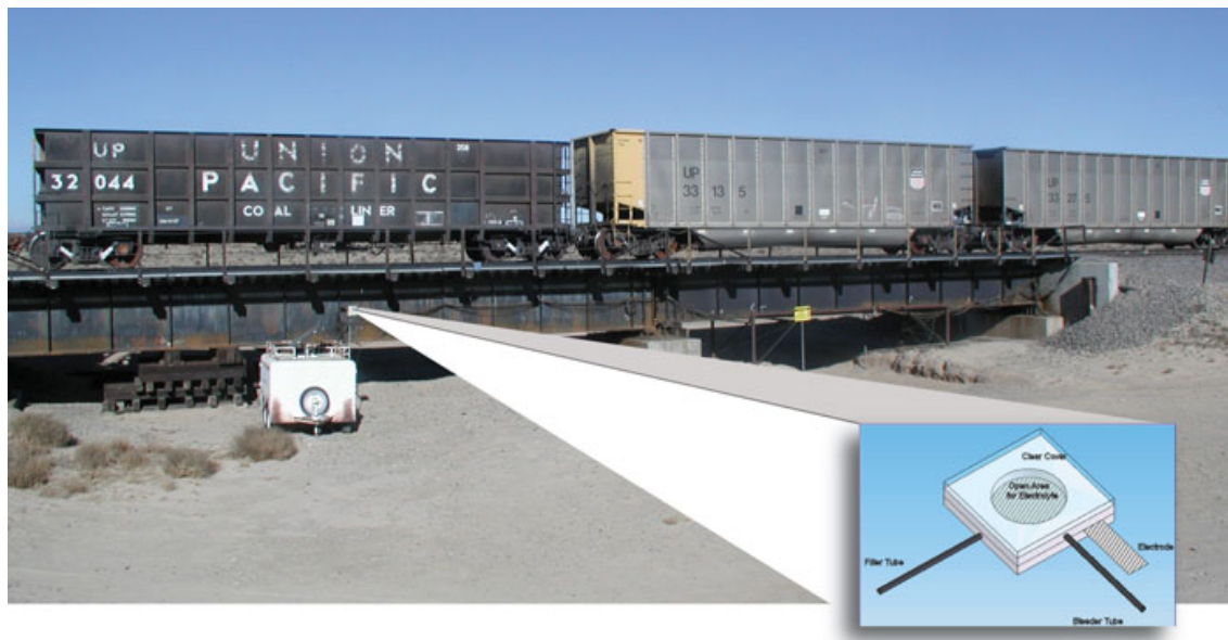
Figure 1. Steel Bridge at FAST
