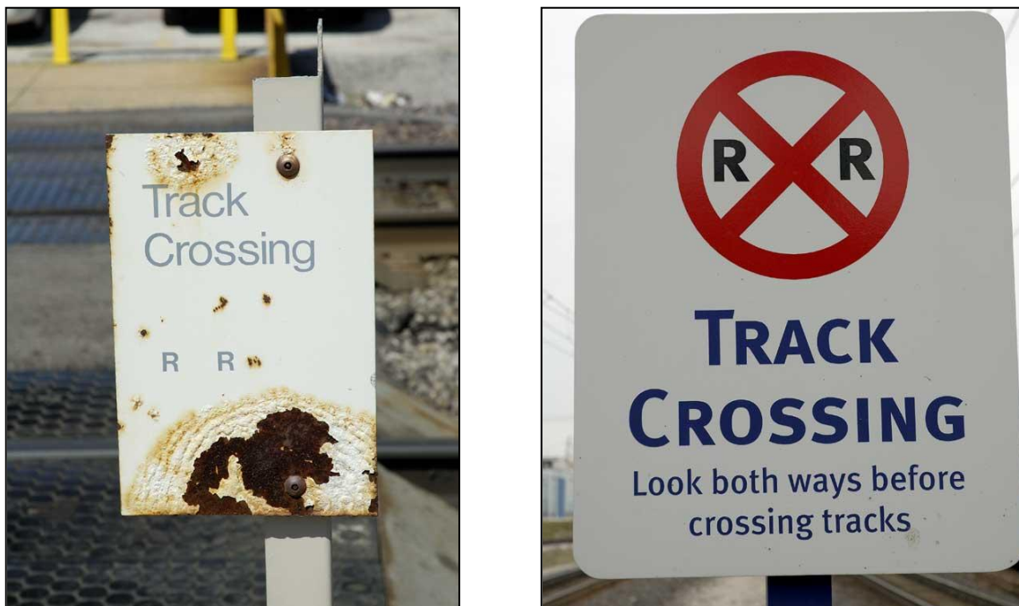
Figure 10: Examples of poor sign maintenance (left) and good sign condition (right).
