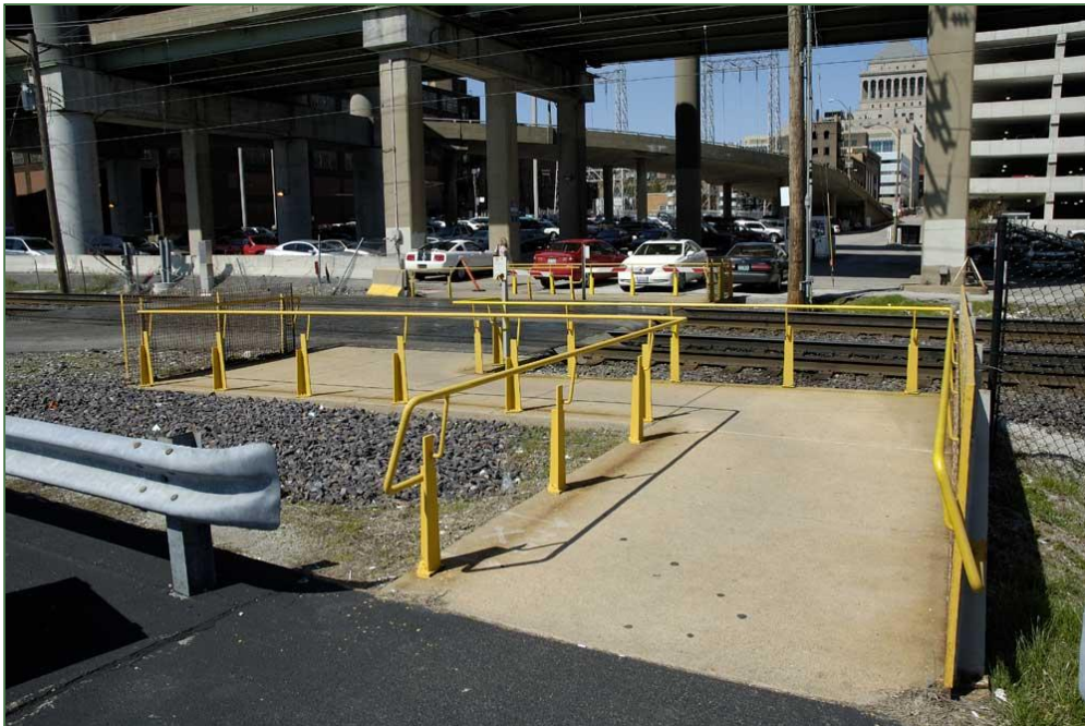
Figure 8: Example of railing used to delineate the desired crossing path for pedestrians.
