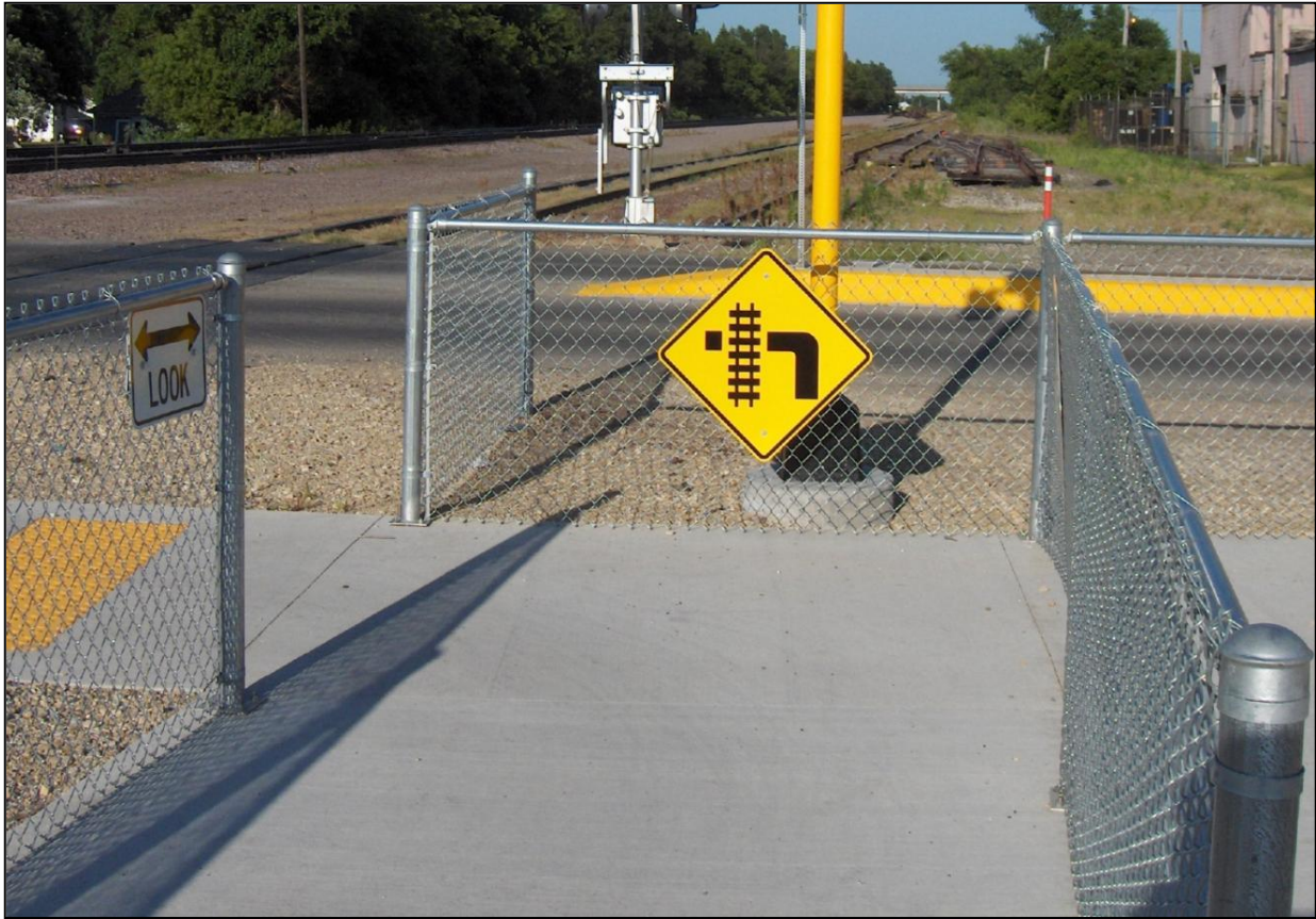
Figure 6: Example of a warning sign combined with right-of-way fencing to channelize pedestrians to the desired crossing location.
