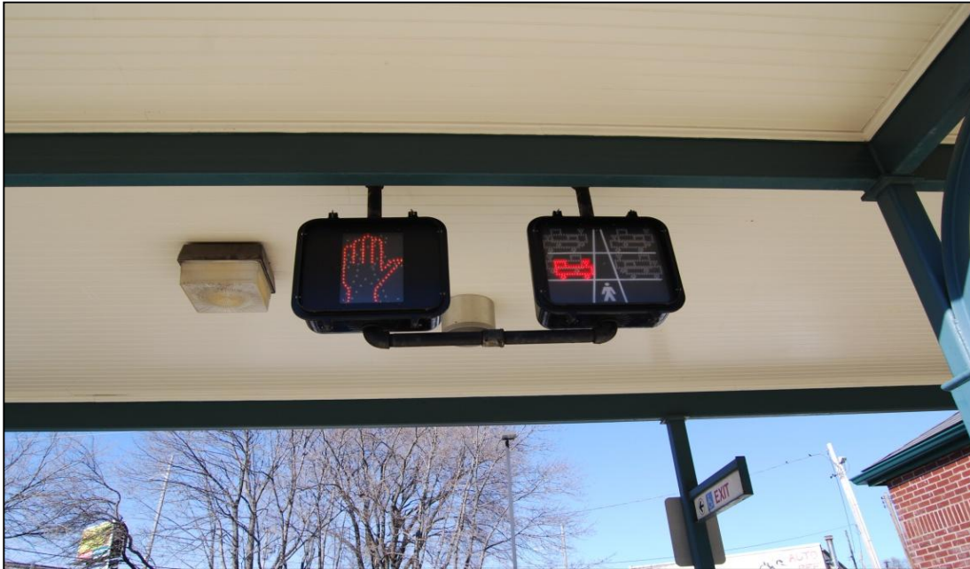
Figure 5: An example of a “Second train coming” display sign used on a passenger station platform.
