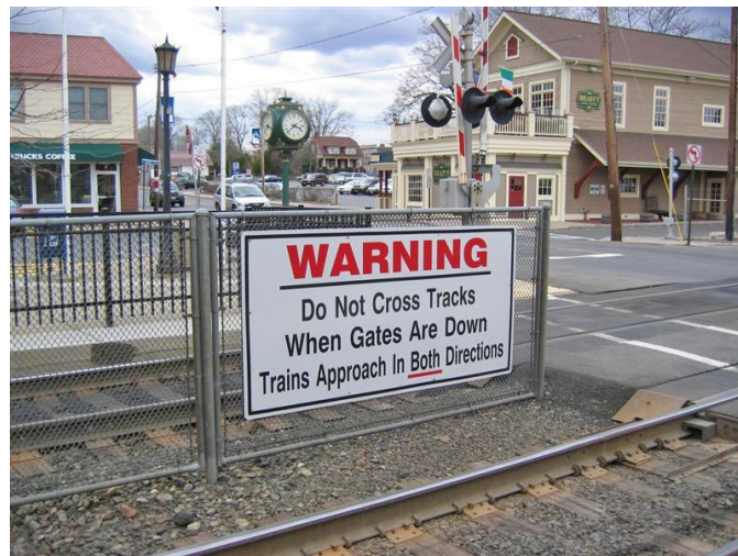
Figure 13: Example of intertrack fencing with warning message posted that clearly indicates both the nature of the hazard, and the intended action to be followed.
