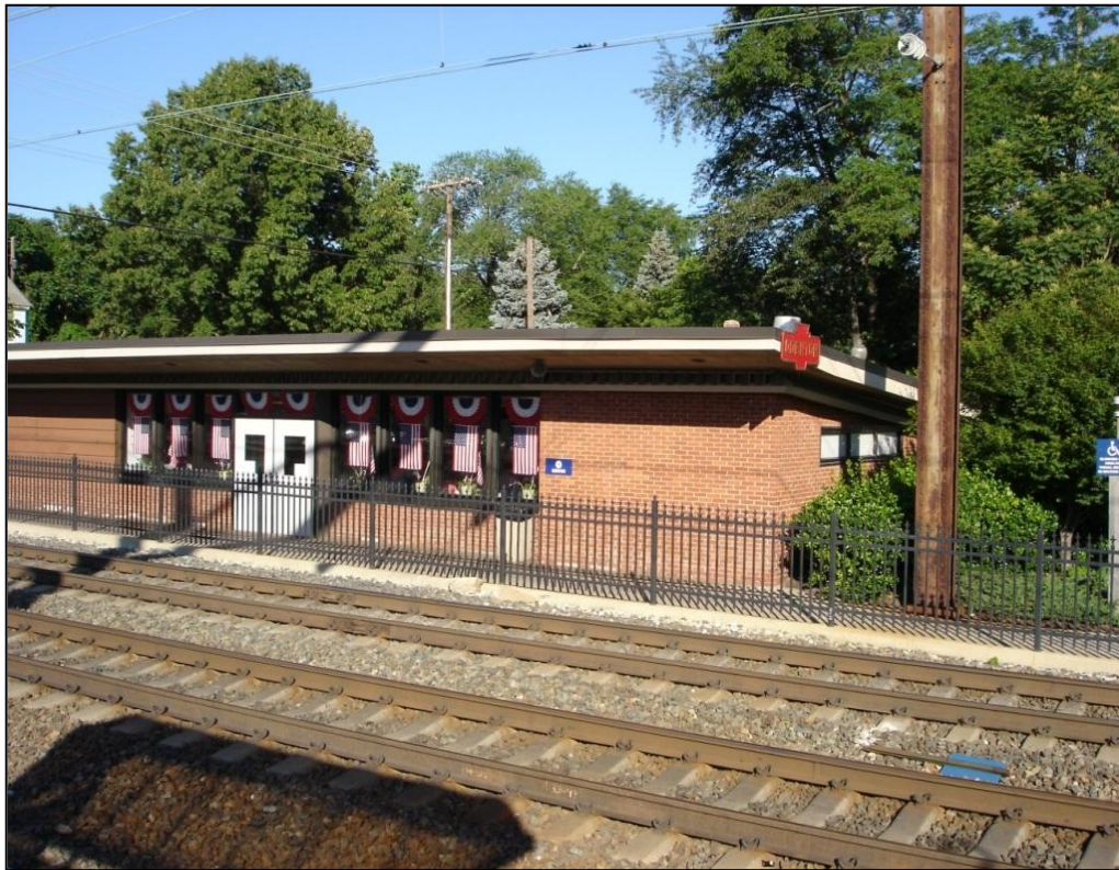
Figure 15: Example of platform edge fencing.
