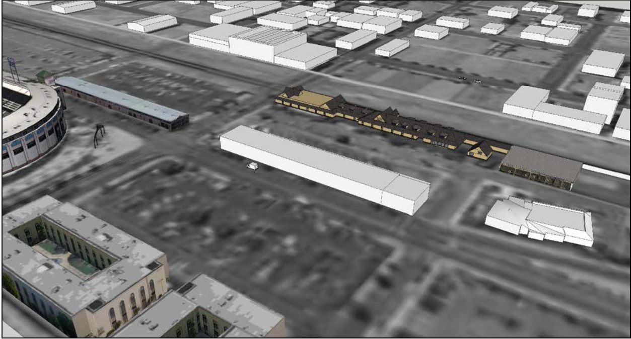
a. South facing aerial view of existing Southern Pacific Railroad Depot.
