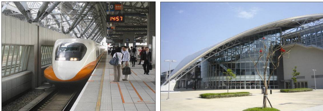
Figure 2-4 Examples of existing stations
