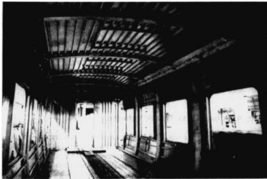
Figure 5-4 Typical Talgo HSGGT Passenger Coach Superstructure
