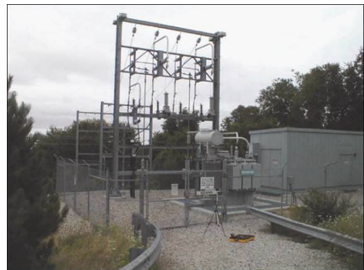
Figure 2-16 Paralleling station
