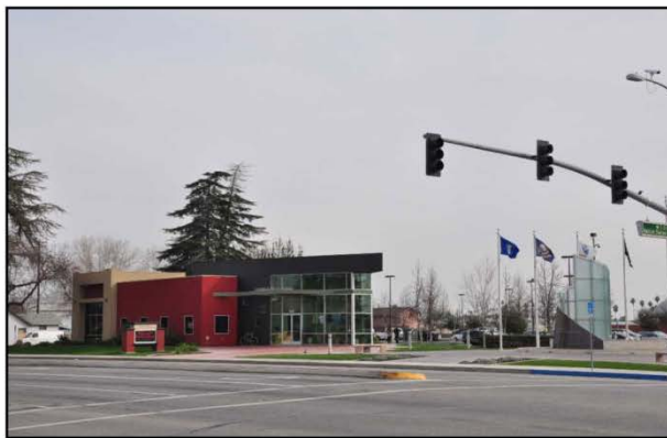
CBD-b. Northern station option from Truxtun Avenue, looking southeast. Station would begin behind building in foreground.
