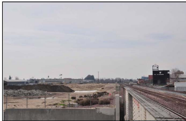
CBI-b. Northern station site option, at alignment, looking west at Union Avenue.
