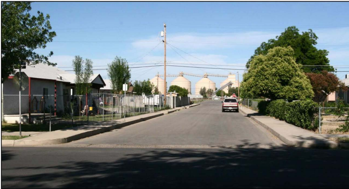
W-b. Alignment from residential neighborhood, central Wasco.
