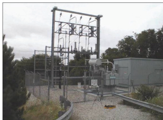
Figure 2-17 Paralleling Station
