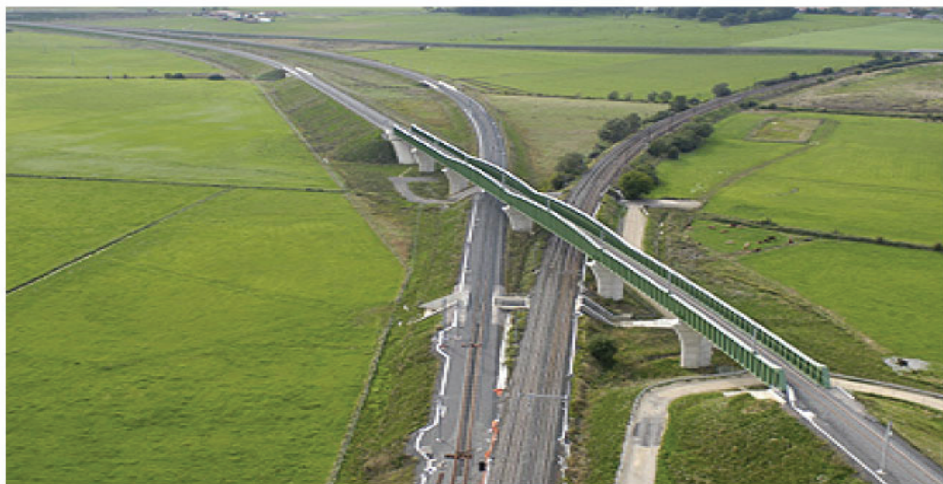
Figure 2-13 Photograph Showing Leg of Wye Crossing over Another HST Track
