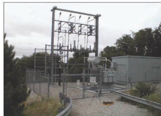
Figure 2-17 Paralleling Station
