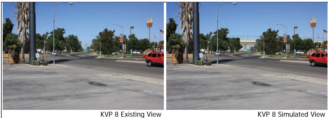
Figure 3.16-10 KVP 8 Existing and Simulated Views Left, Existing View: View to the northeast from the Downtown Chowchilla gateway. The SR 233–SR 99 interchange is visible in the center of the view. Right, Simulated View: The elevated HST guideway would appear across the center of the view, above the SR 99–SR 233 interchange.
