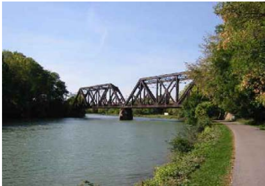
Figure 2. Pittsford, NY, railroad bridge chosen for demonstration project
