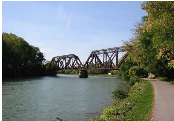
Figure 2. Railroad Bridge Chosen for Demonstration Project
