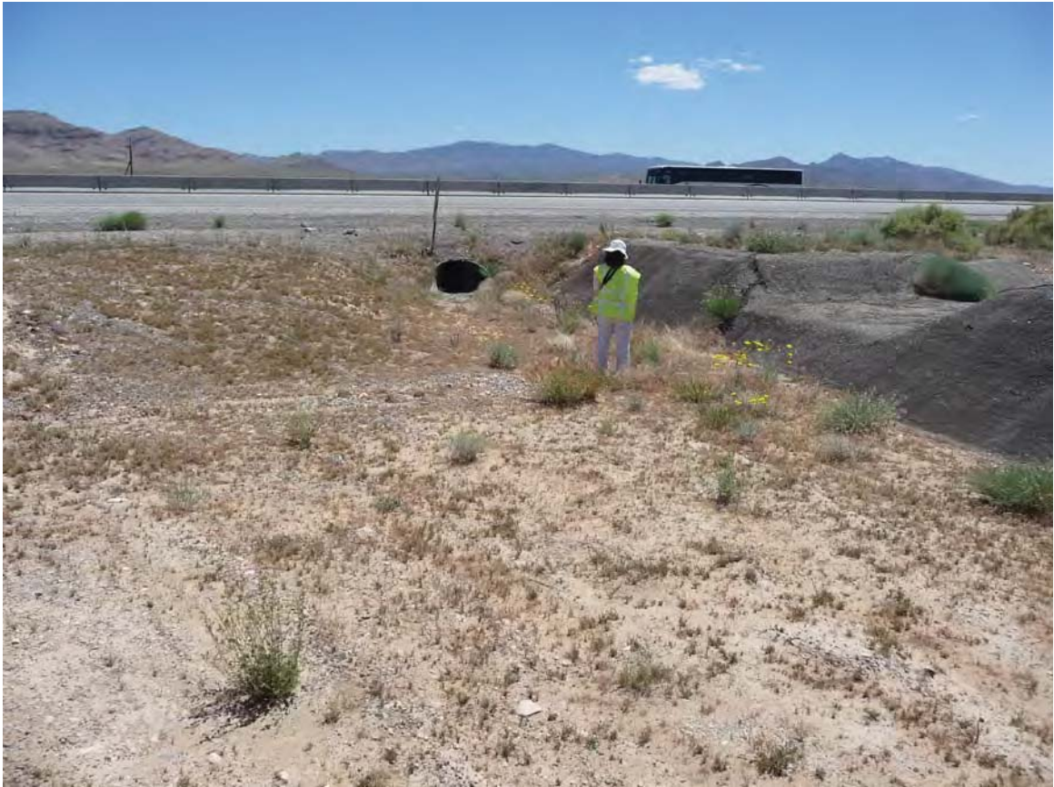
Exhibit A. Figure 31. Manmade drainage connecting to road culvert within HUC 8 Ivanpah-Pahrump Valleys Watersheds / HUC 12 Town of Jean -Frontal Ivanpah Lake Subwatershed
