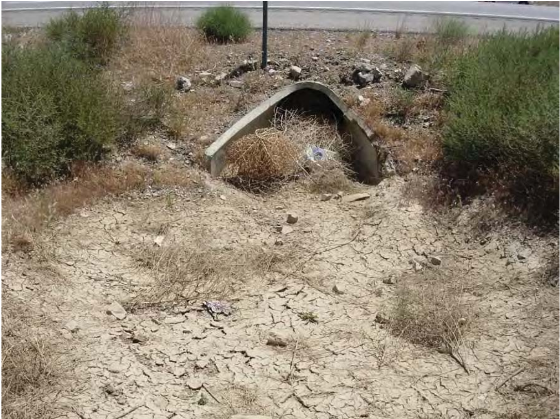
Exhibit A. Figure 15. Manmade drainage connecting to road culvert within HUC 8 Ivanpah-Pahrump Valleys Watersheds / HUC 12 Ivanpah Subwatershed
