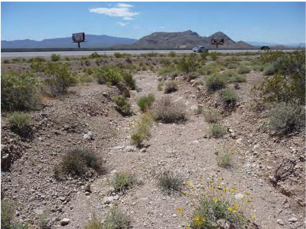
Exhibit A. Figure 32. Manmade drainage connecting to road culvert within HUC 8 Ivanpah-Pahrump Valleys Watersheds / HUC 12 Town of Jean -Frontal Ivanpah Lake Subwatershed
