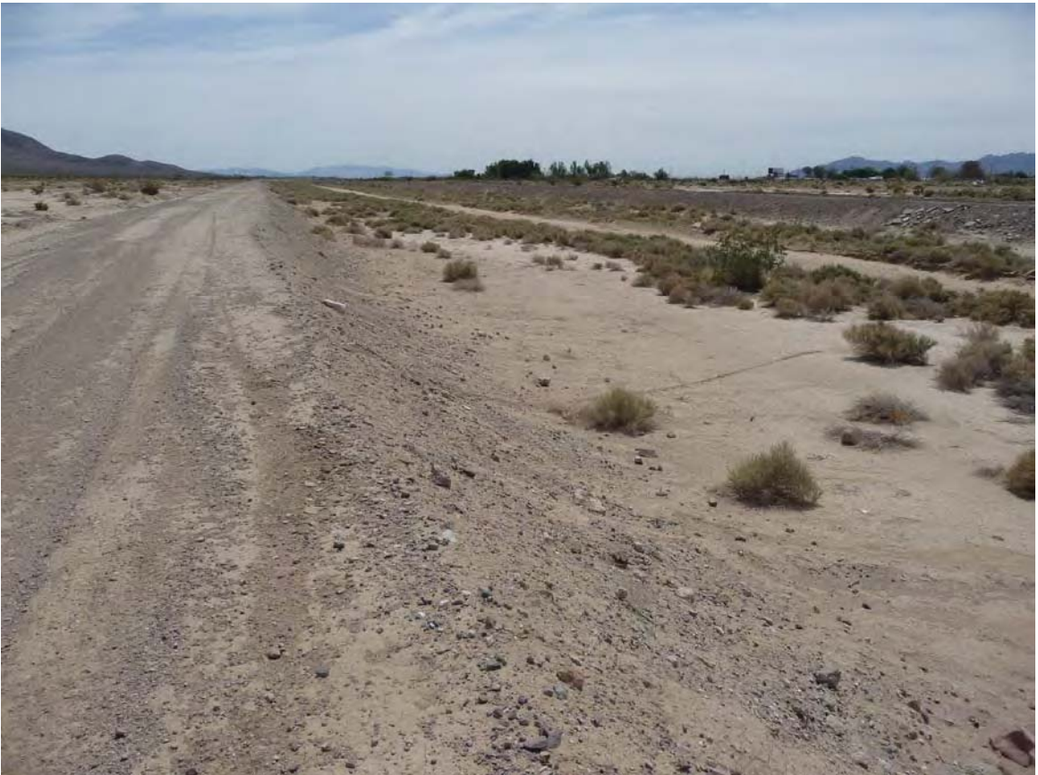
Exhibit A. Figure 32. Manmade drainage connecting to ephemeral drainage within HUC 8 Mojave / Coyote-Cuddeback Lakes Watersheds / HUC 12 Halloran Spring-Halloran Wash Subwatershed
