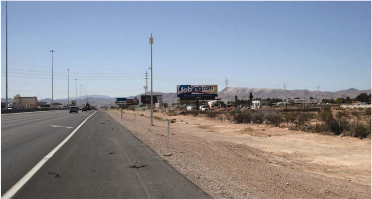
Existing View from Westbound I-15 of Las Vegas MSF Option 1 (Wigwam Avenue) Site
