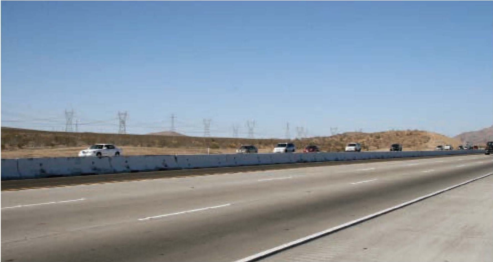
Existing View from I-15 Eastbound of Victorville OMSF Site 2
