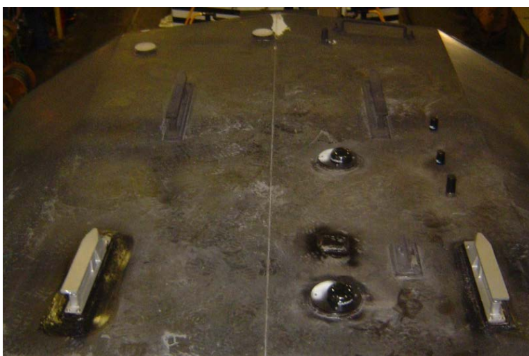
NS 2623 Rooftop View Figure 3b
