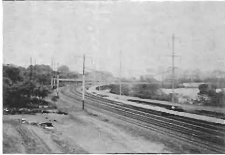
54th STREET and ARSENAL RETAINING WALL
