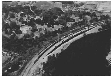
54th STREET and ARSENAL RETAINING WALL
