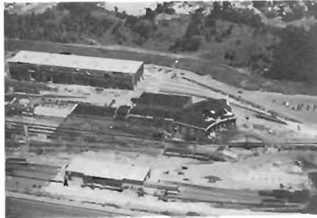
REPAIR SHOP and ANNEX BUILDINGS
