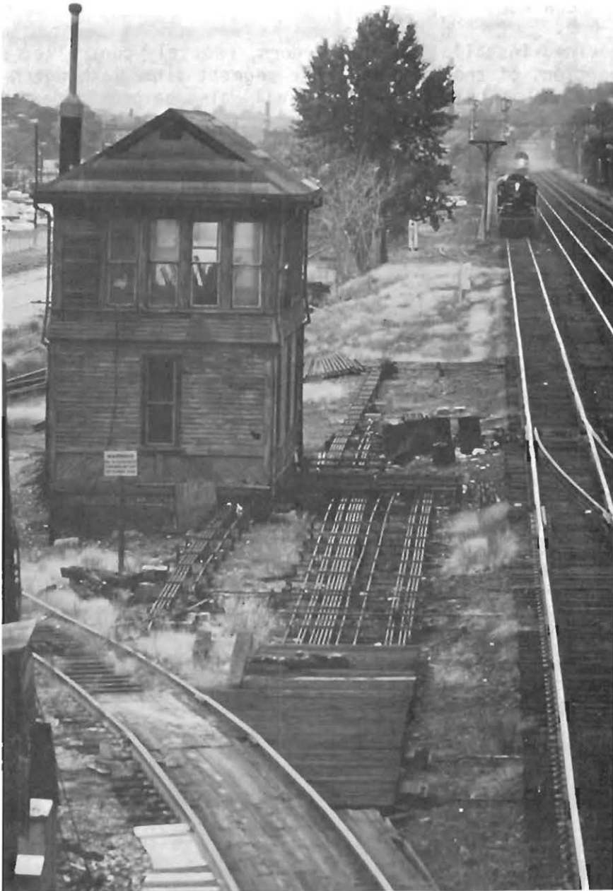
Hand-operated interlocking connected to switches by pipes, vintage 1906. The NECIP converted some, but by no means all, of these antiquated facilities to modern electric operation.
