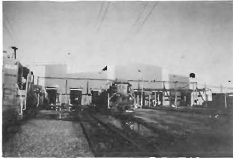
NEW ROOF and SIDING LOCOMOTIVE BUILDING
