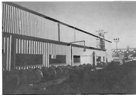
NEW ROOF and SIDING, WHEEL BUILDING
