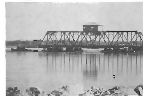
FLOAT IN OF SWING SPAN
