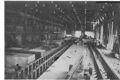
INTERIOR REPAIR SHOP SHOWING FIRST THREE TRACKS
