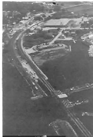
NEW SWING SPAN
