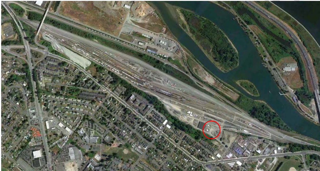
BNSF Delta Locomotive Yard Figure 1
