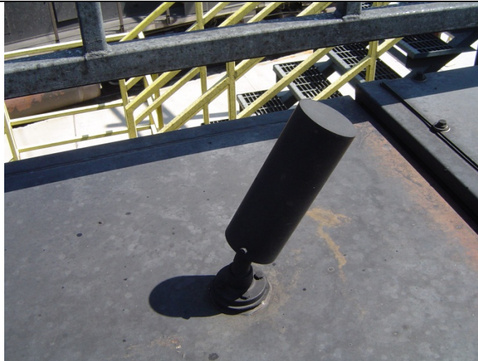
Damaged VHF antenna Figure 36
