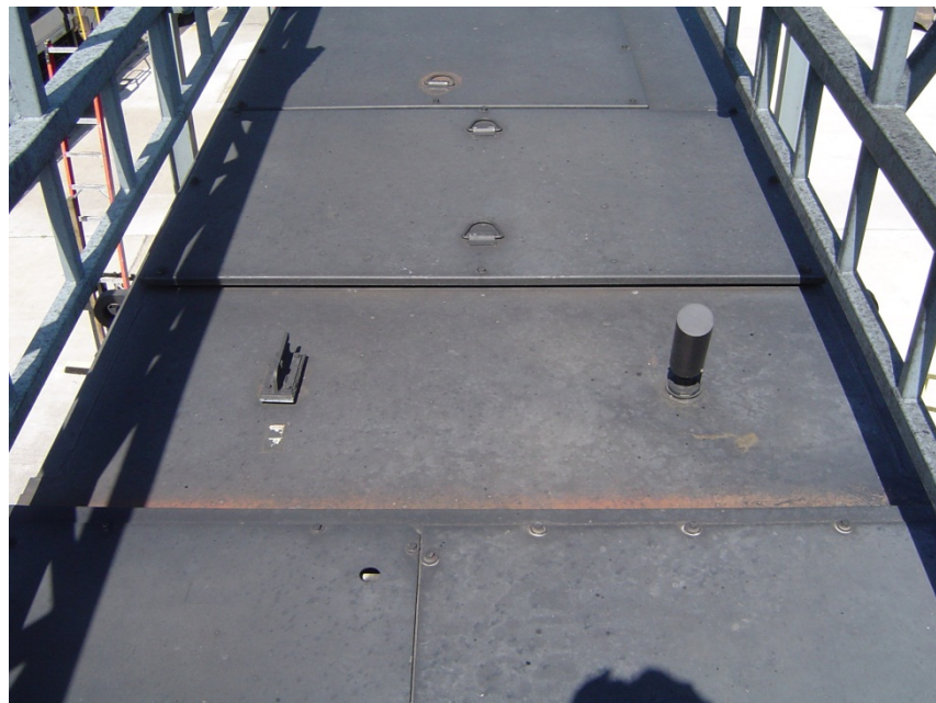
NS 8898 Rooftop View Rear Facing
