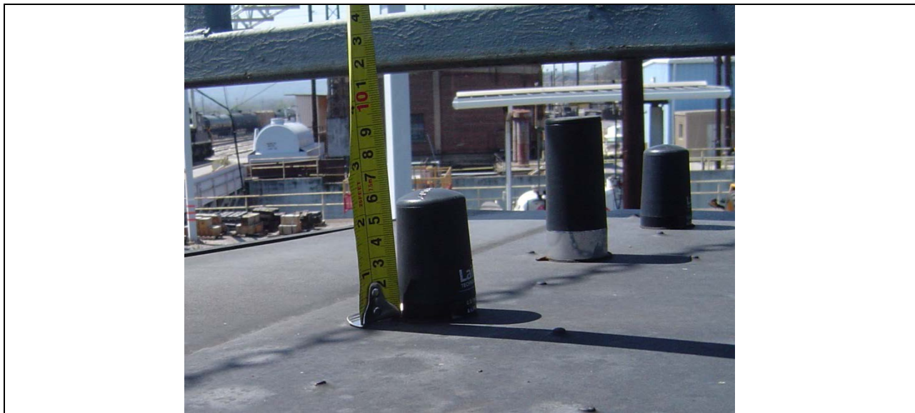
Center antenna is designated as 802.11 According to physical height >3" it can only be in the cellular range MLPV-698 Figure 38
