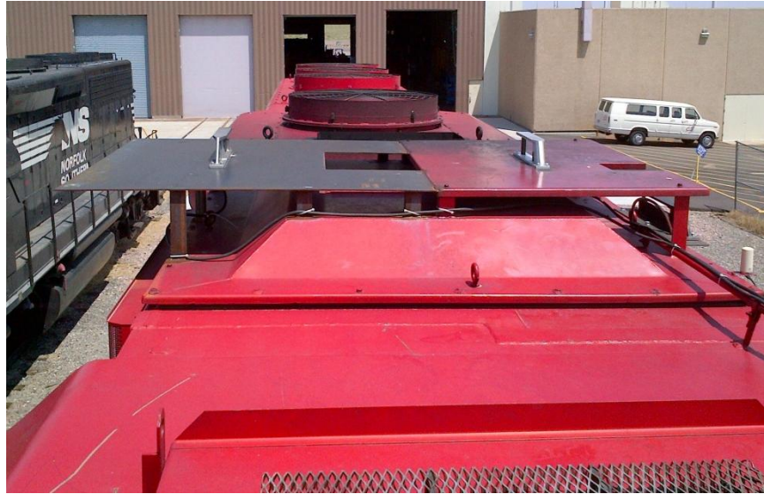
Figure 18: Typical locomotive 220 MHz antenna install
