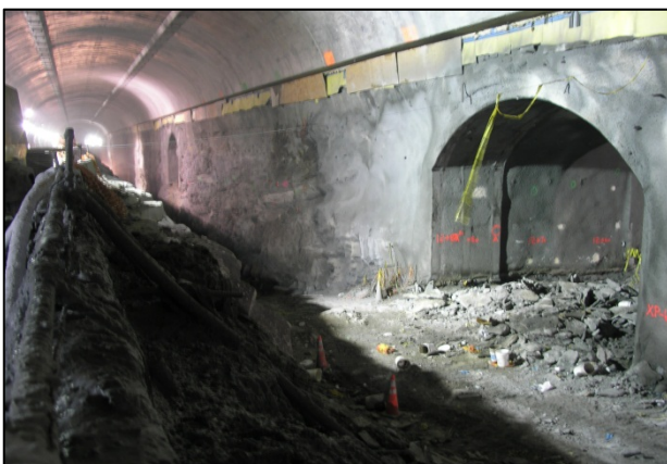
Manhattan: Tunneling at Mezzanine-Level Showing a Cross-Passage
